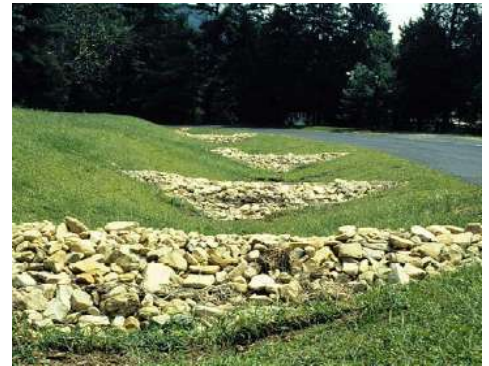
Stone check dams slow the flow of water.
