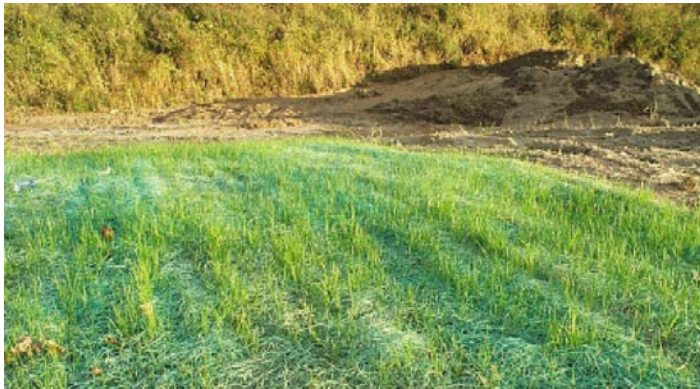
Figure 5.4. Exposed slope stabilized with erosion control matting
