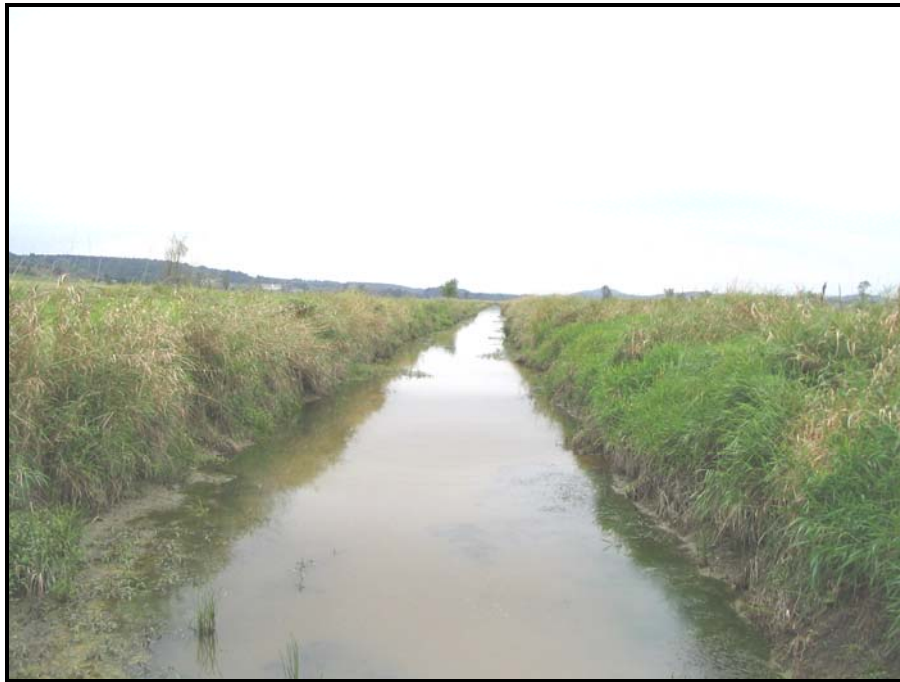
Figure 2: Constructed ditch draining agricultural fields within the floodplain of the Lemon Fair River. During high flow events, runoff and associated P flows through adjacent fields, into the ditch and ultimately discharges into the Lemon Fair River.
