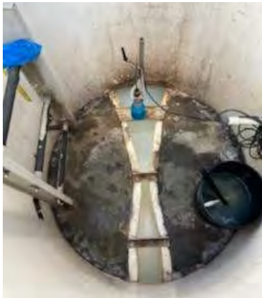
Figure 2. Commonwealth manhole and flume.
