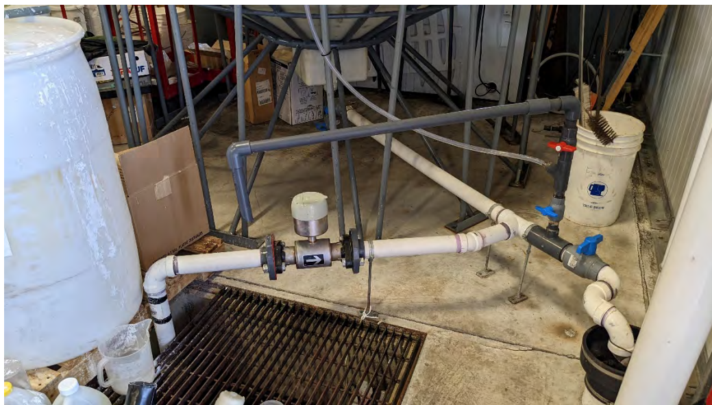
Figure 14. Effluent pipe and grab sample location at Rock Art.
