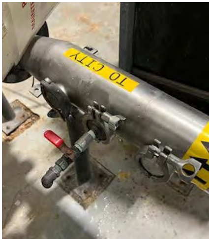
Figure 3. Grab sample collection point on effluent line.
