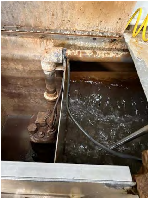
Figure 11. Equalization tank at VT Precision.
