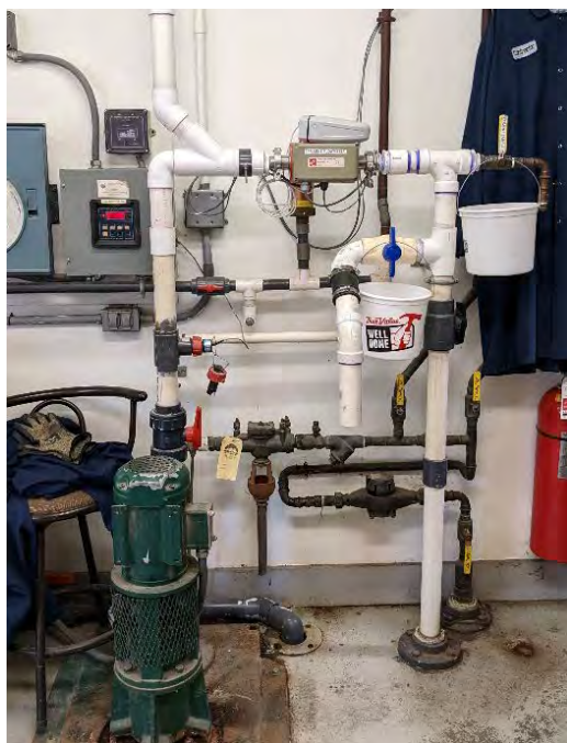
Figure 6. Ben & Jerry's - Waterbury discharge pipe with inline flow meter.
