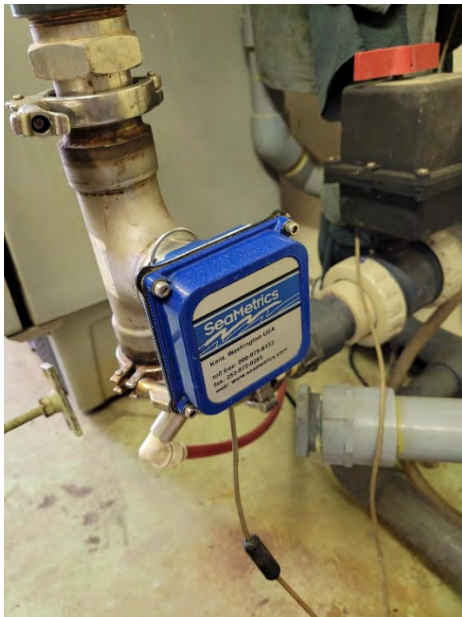
Figure 10. Zero Gravity Brewery discharge pipe with inline flow meter.
