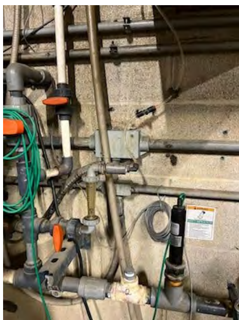
Figure 4. Discharge pipe with inline rotimeter for triggering autosampler and pH meter for pH measurements.
