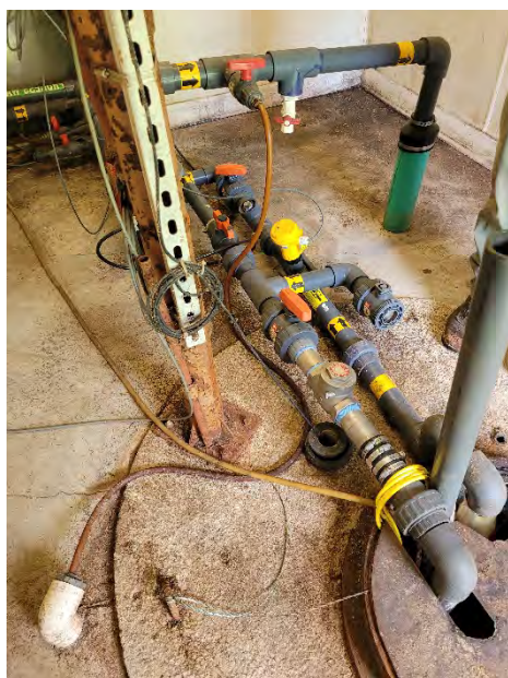
Figure 2. Otter Creek Brewery discharge pipe with inline flow meter.
