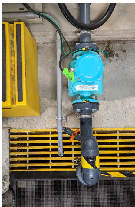
Figure 2. Grab sample collection point on effluent line and grate leading to composite sample intake line location.
