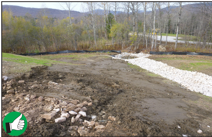
After installing rock outlet protection
