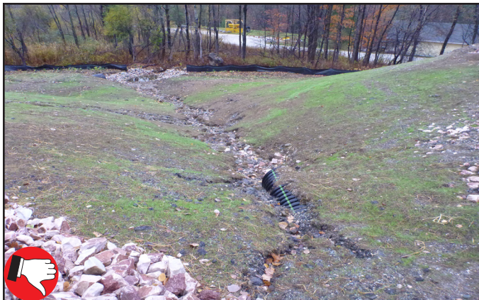
Before installing rock outlet protection
