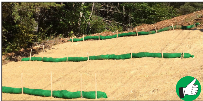
Good use of filter socks along a slope to slow runoff velocity.
