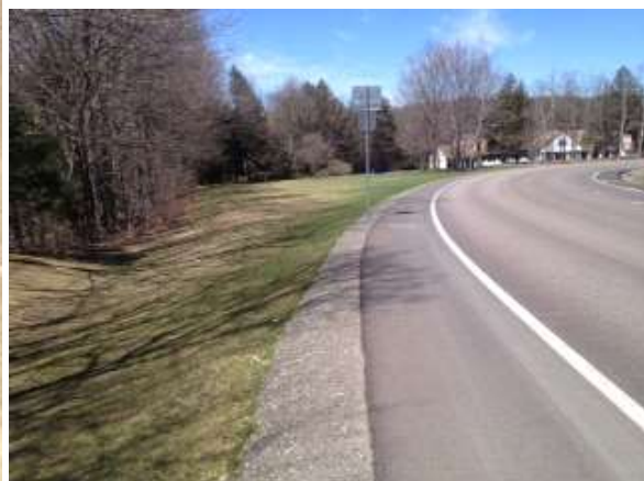
Example of distributed flow, low shoulder
