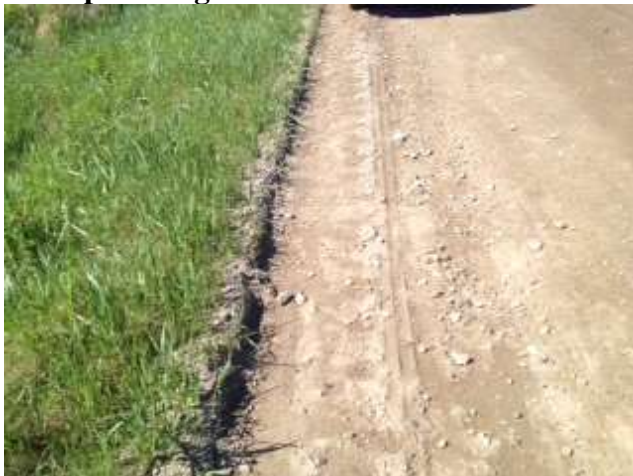
Example of high road shoulder
