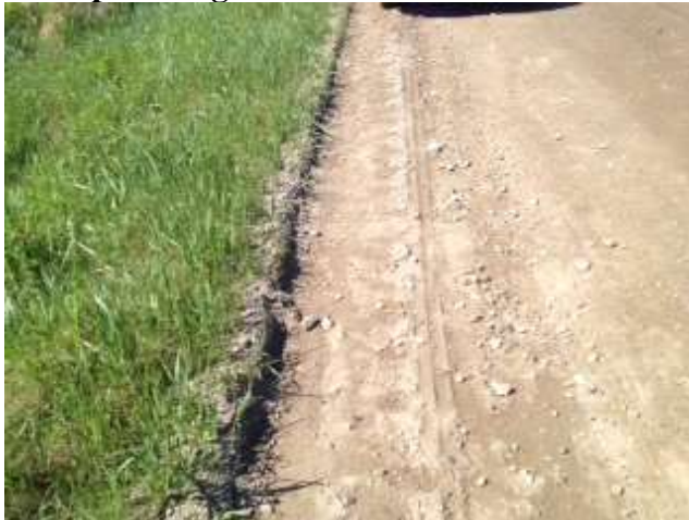
Example of high road shoulder
