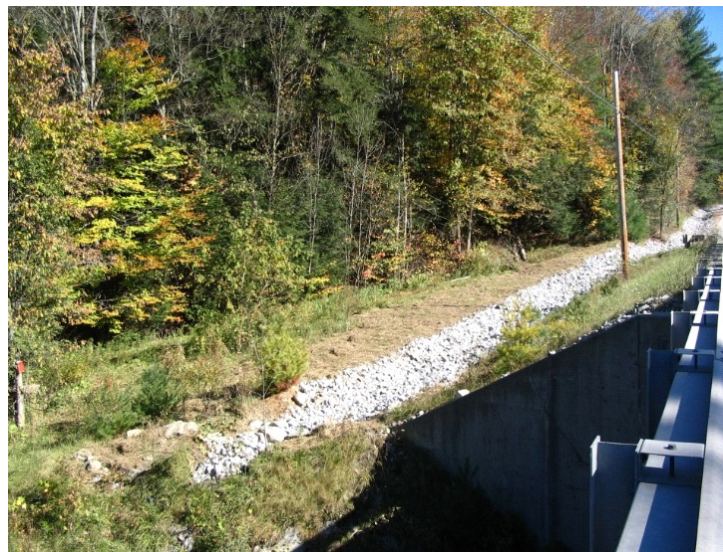
Example of an armored turnout at a hydro bisect site
