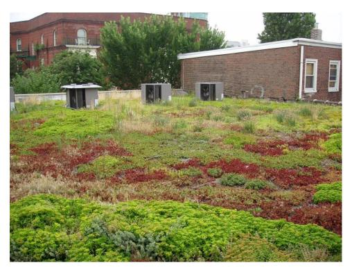
Figure 4-22. Example of Extensive Green Roof, Philadelphia, PA, Design Guidance (Source: UNHSC)
