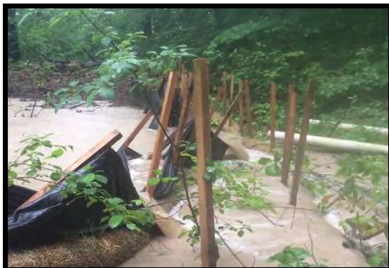
This silt fencing was not properly maintained, resulting in failure and discharge of polluted stormwater to the City's waterways.
