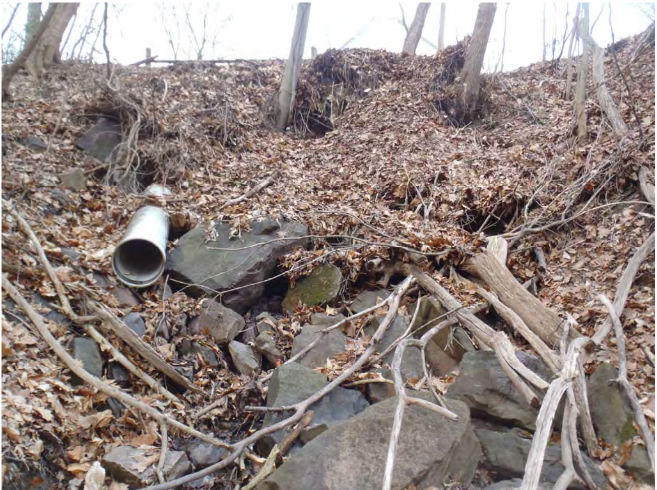
Photo 5: Large Stone Rip-Rap at Outfall
