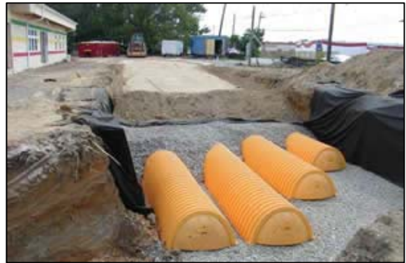
Figure 6. An underground storage system CR: http://www.stormtech.com/images/pic_engineer.jpg
