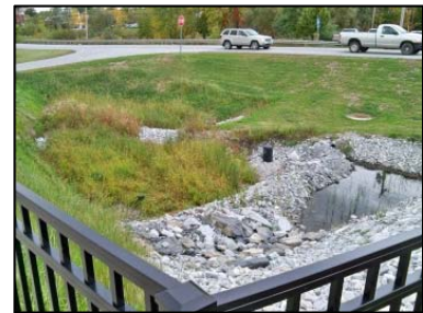
Figure 1. Gravel Wetland at St. Albans Park & Ride
