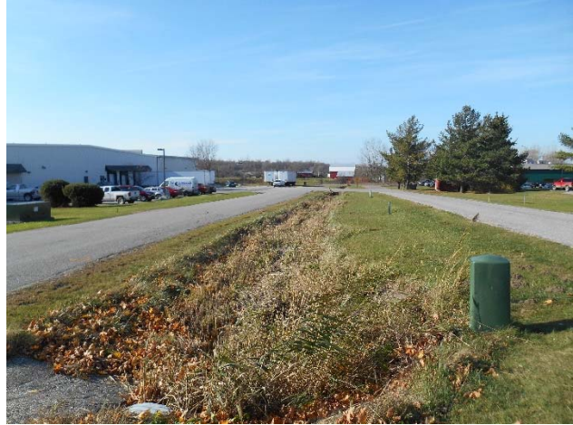
Figure 3. Industrial Park median swales which drain to the area of the proposed new detention pond.
