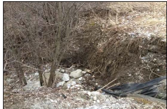
Figure 15. Eroded embankment by Grice Brook Retirement Community
