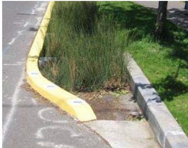
Figure 14. Example of a stormwater curb extension for the Route 7 ROW (Credit: VA DRC Stormwater Design Manual 2013).
