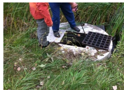
Figure 2. WCA and Town Public Works Director inspect #3410-9010 outlet structure to verify pond routing.
