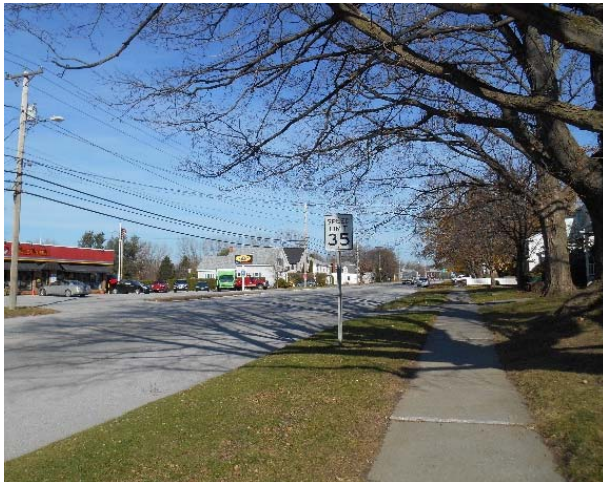
Figure 13. Site for "M1" Stormwater Curb Extension along Route 7.
