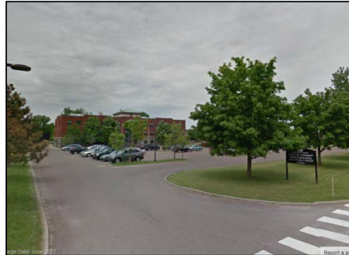
Figure 12. Project site by the State’s facility on Houghton Street
