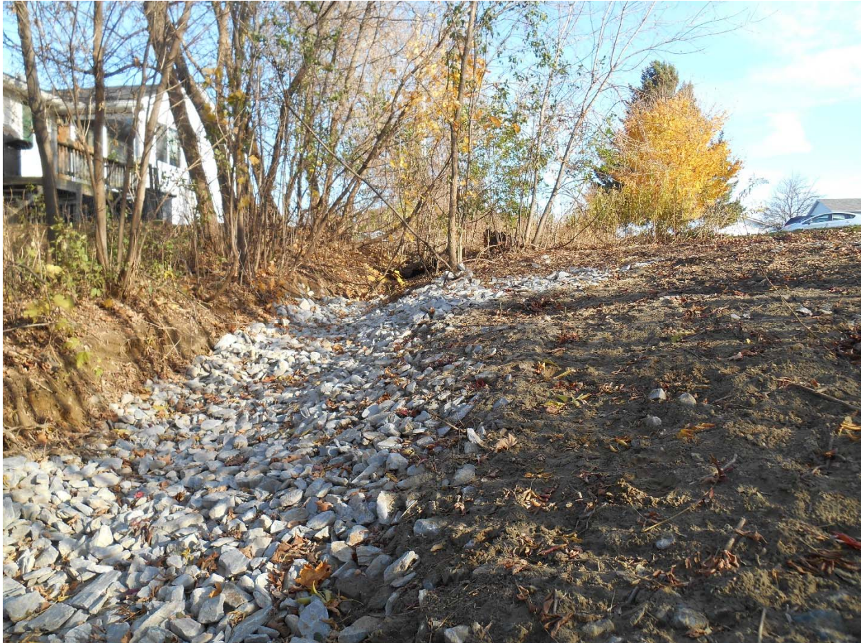
Figure 8. New stone cover in existing drainage swale, near location of the new infiltration basin.
