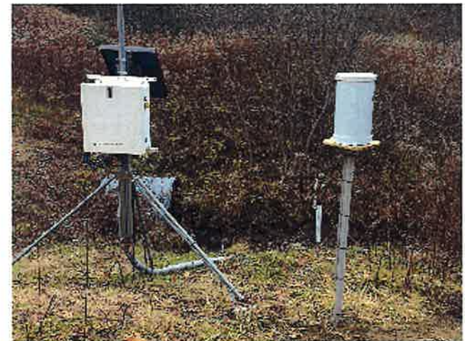
Streamflow and precipitation monitoring station at Sunderland Brook.
