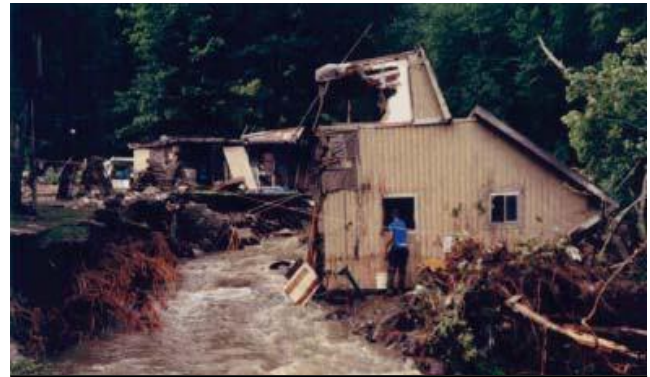
Catastrophic erosion during the 1990 flood, Great Brook, Plainfield, VT
