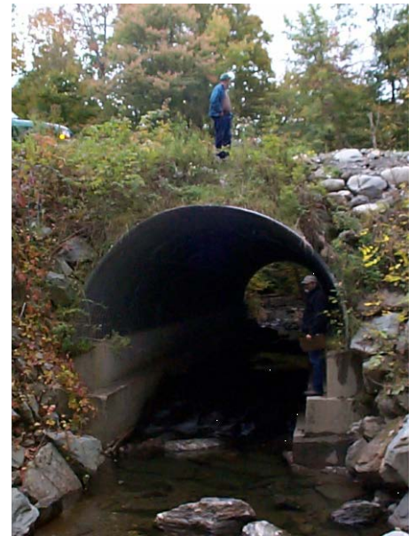
Figure 8. Stepped footers on an arch.
