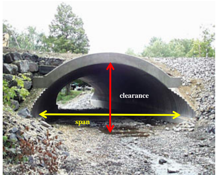
Figure 2. Measuring arch span and clearance.
