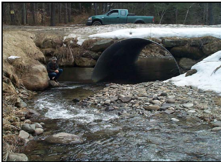
Figure 5. Steep riffle spanning the channel cross-section immediately upstream of the structure opening.
