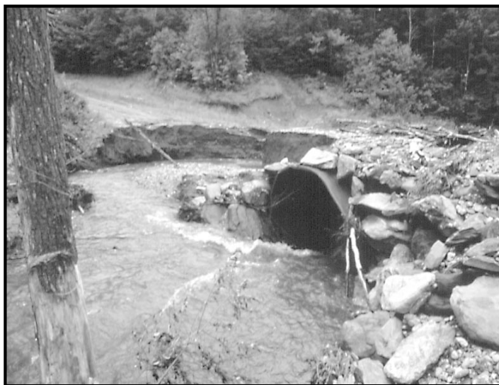
Figure 11. Outflanking Failure at undersized culvert where upstream sediment deposits were observed.
