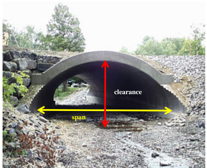
Figure 2. Measuring arch span and clearance.
