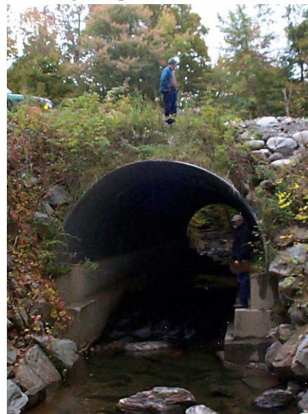
Figure 8. Stepped footers on an arch.
