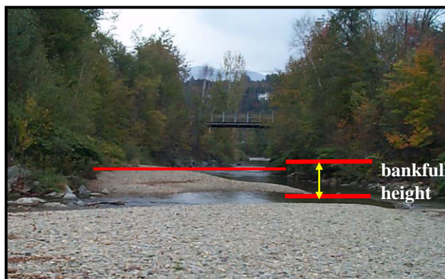
Figure 9. Example of sediment deposit upstream of an undersized bridge that has built to an elevation greater than \frac{1}{2} the bankfull height.
