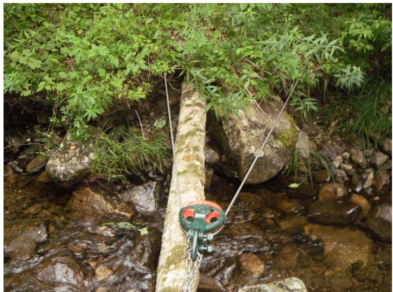
Figure 22. A pulley can be used to increase force when driving a spear into the bank.
