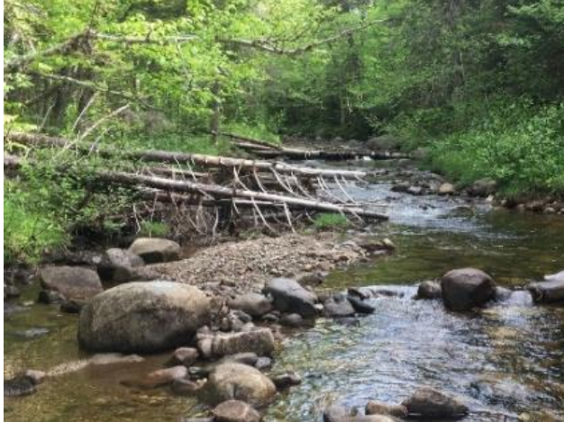
Figure 20. The tops of these spruce trees were cut to prevent the river from snapping them.
