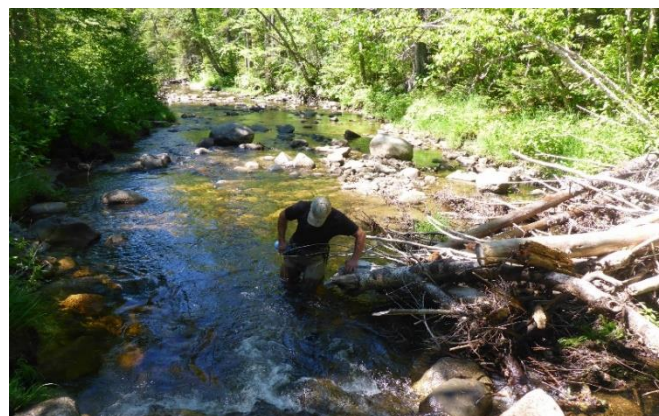
Figure 8. This reach responded rapidly and dramatically to strategic wood addition because of a high bed load and ideal combination of slope and width.
