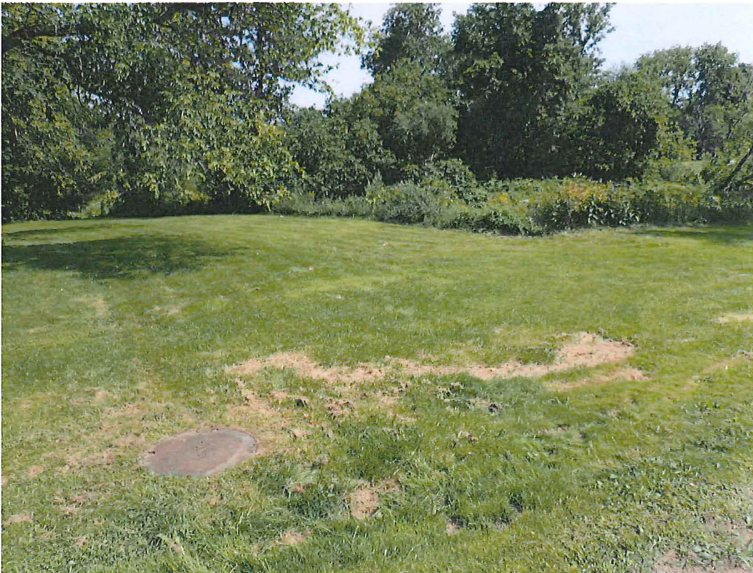
Photo 4. This is the sewer manhole that will be the connection point for the proposed force main. (August 24, 2016)
