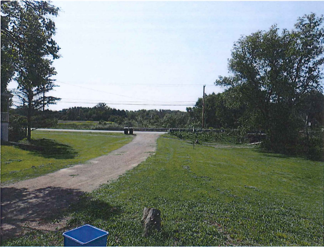
Photo 1. View to the south towards Williston Road from the pump station. The house is just off the left edge of the photo. The proposed force main would run to a directional boring staging area in the lawn and then angle to the right and cross the brook just this side of the tree at the right side of the photo. (August 24, 2016)
