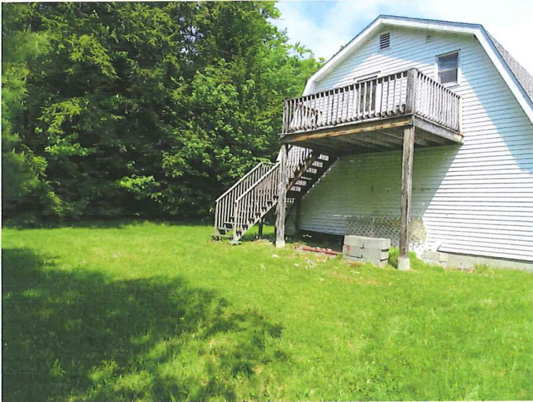
Back of garage with apartment above
