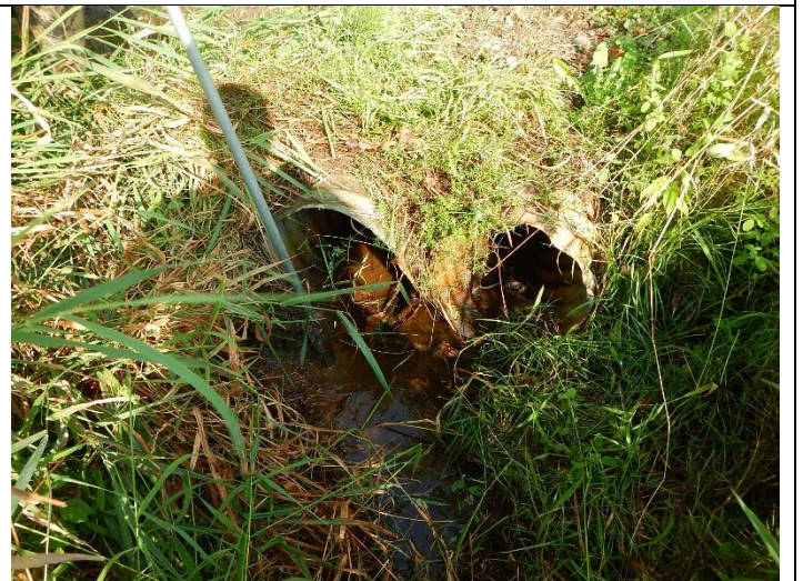
Photograph 10. Culverts under access road crossing of 2015-JD-1
