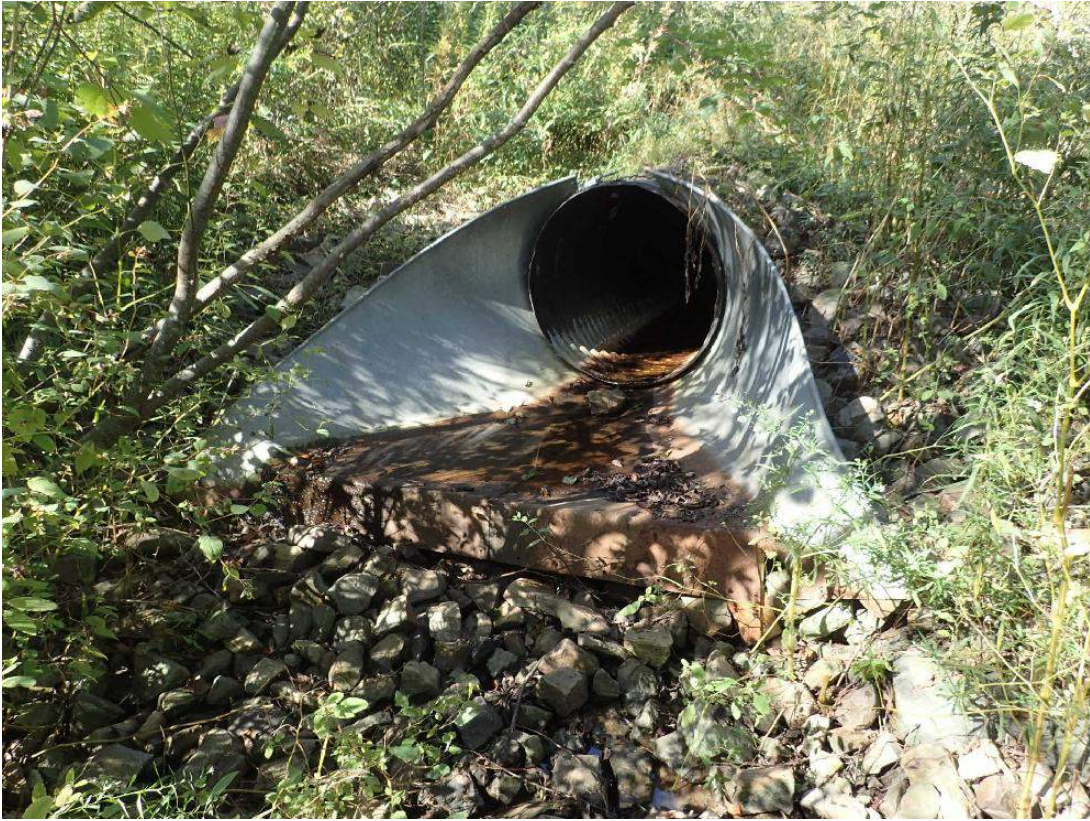
Photo 1. Outfall of existing culvert from stormwater basin (September 27, 2016)
