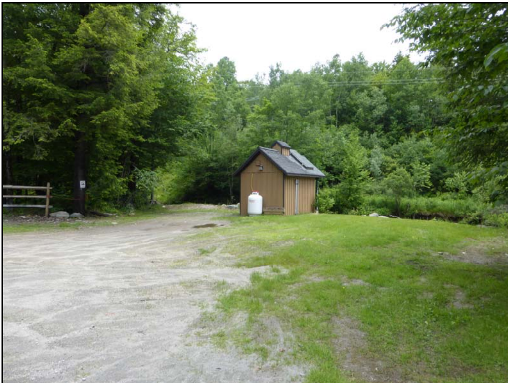
Photo 4. Photo shows the pump house structure near where the sewer force main is to be installed across the Cold Brook. View is to the east.
