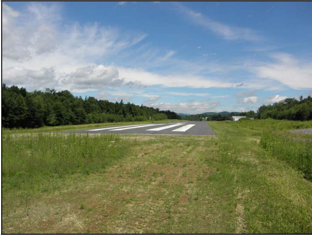
Photo 9. Photo shows the southern end of the runway at Deerfield Valley Regional Airport. View is to the north.
