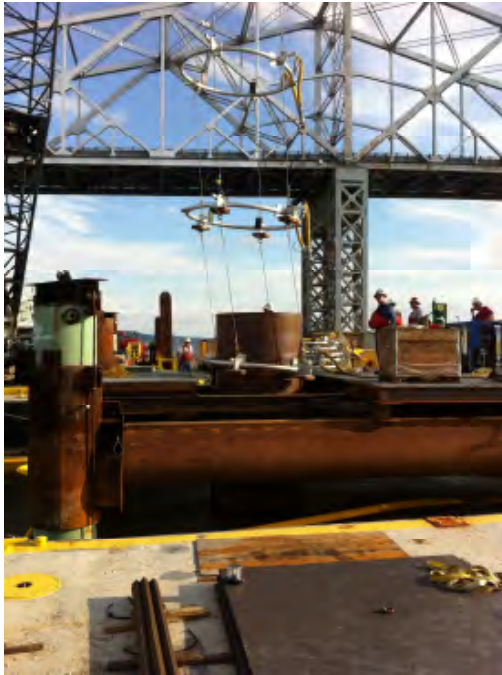
Figure 3. Deployment of the Unconfined Multi-tier Bubble Curtain
