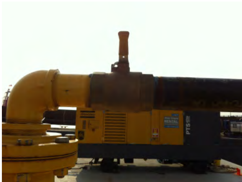
Figure 7. Valve at the Reservoir Tank Inlet
