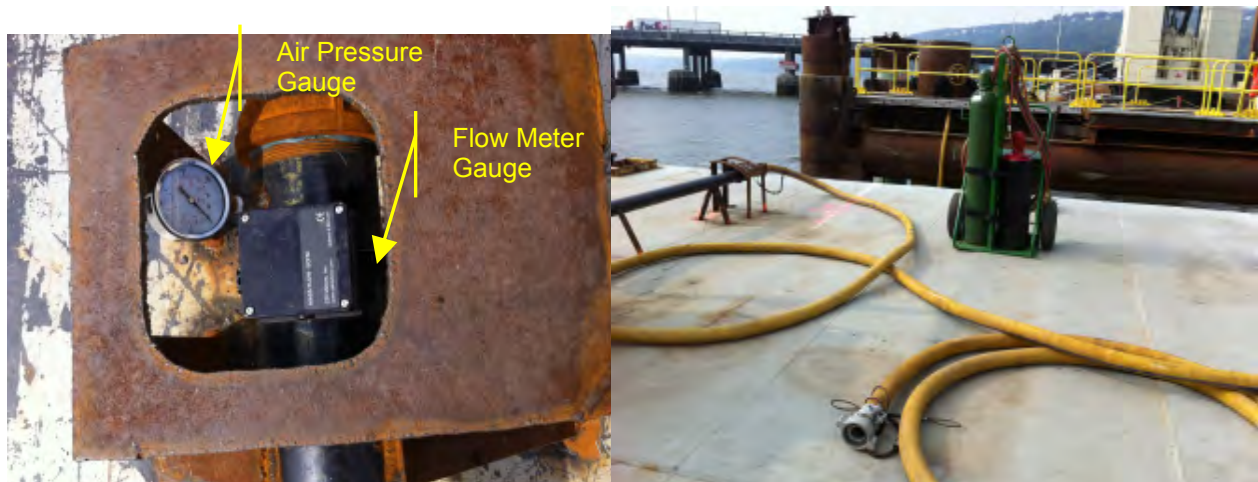
Figure 2. Flow Meter and Pressure Gauge on Outlets from the Reservoir Tank to the Bubbler Ring
