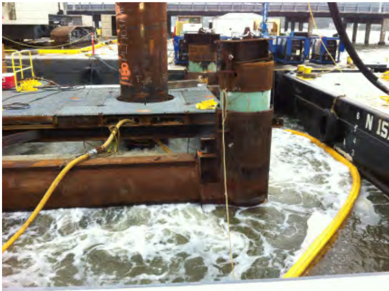
Figure 4. Operation of the Multi-tier Bubble Curtain
