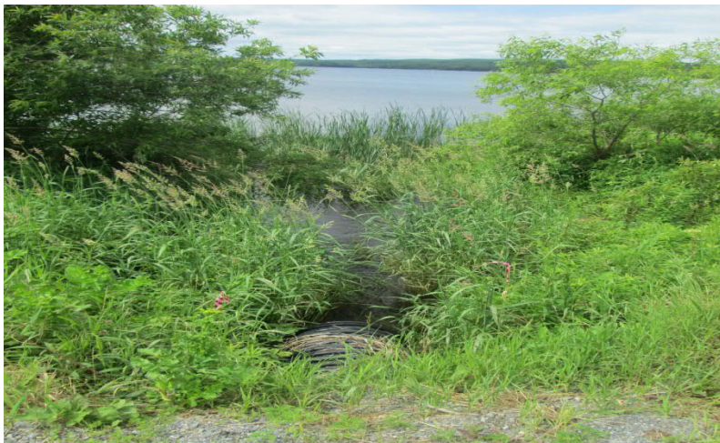
Culvert Outlet, South Side
