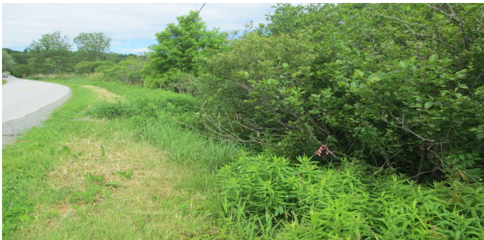
Culvert Inlet and Wetland, North Side
