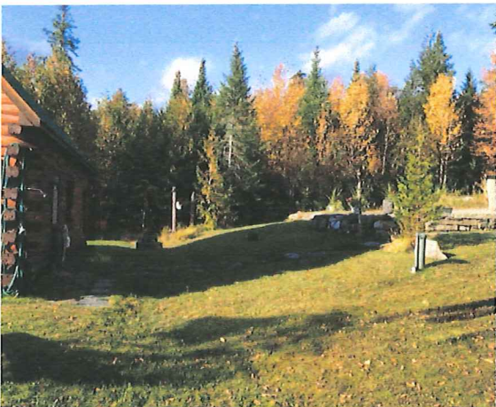
Rear of main cabin where addition and porch will be constructed.
