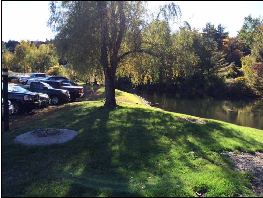
Photo 1: View southwest of the detention pond from the edge of the existing parking lot.
