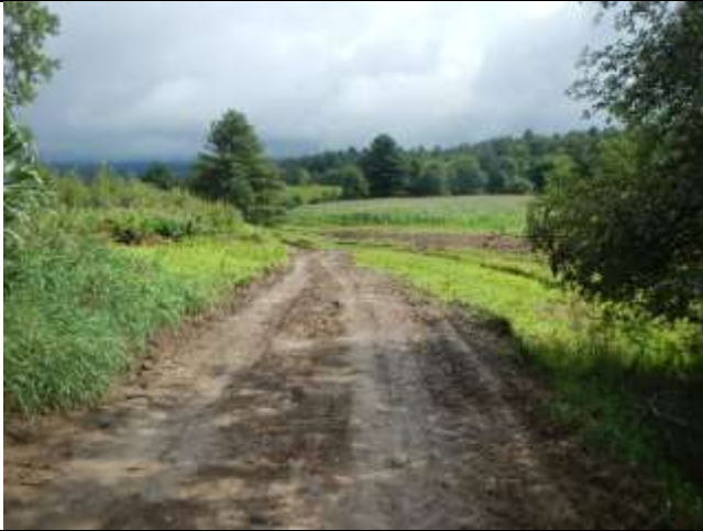
Photograph 3. Looking down the existing access road, view to the northeast with laydown area to the left and array area to the right in the background.
