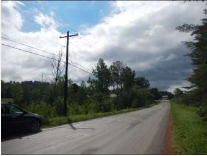
Photograph 1. Looking south along Silver Ridge Road from the end of the existing Project access road; aerial 3-phase line in view.
