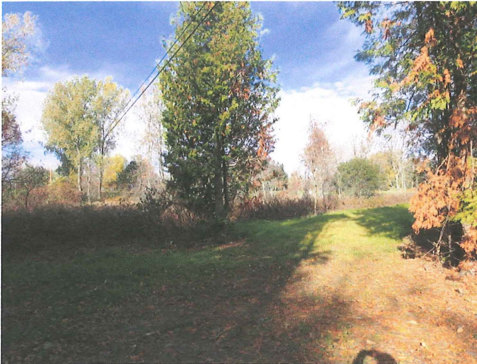
Photo 4: Forcemain crossing under power line north of Lot #1 view to the northwest.
