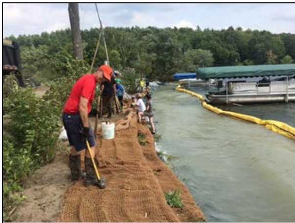
Figures 3 and 4. Example of GSI project in Castleton at Cedar Mountain Road (“encapsulated lift project” to stabilize the road and provide for natural shoreline erosion control)
