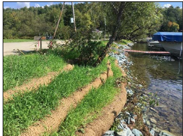
Figures 3 and 4. Example of GSI project in Castleton at Cedar Mountain Road (“encapsulated lift project” to stabilize the road and provide for natural shoreline erosion control)
