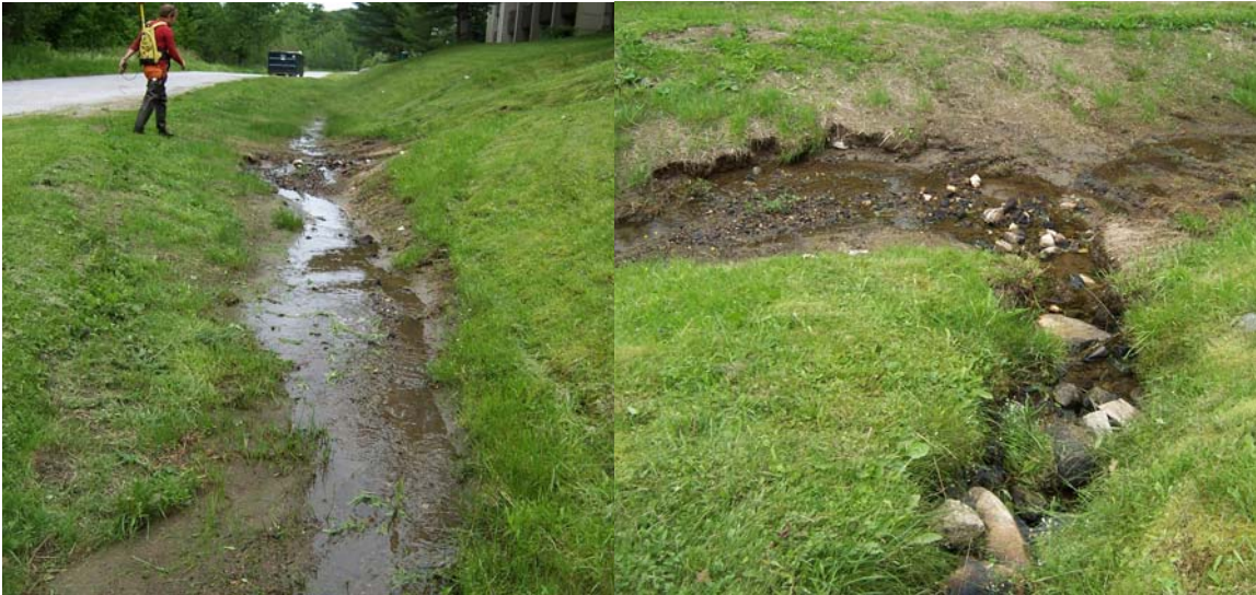
Photographs 49 and 50: A sediment filled tributary to Roaring Brook was followed upstream and ended in this eroding swale at the north corner of the Pinnacle Condos.
