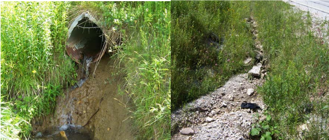
Photograph 14 and 15: On the east side of the Access Road, a rusted out perched culvert and gravel filled swale is conveying sediment into a small tributary of Roaring Brook.
