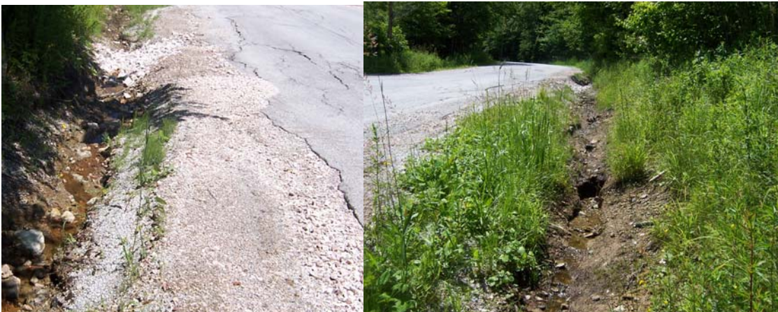
Photograph 29 and 30: Instable and eroding swale has clogged a culvert and is contributing sediment to Ram’s Head Brook.
