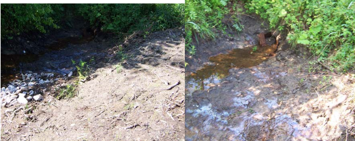
Photographs 8 and 9: The banks around the outlet of a culvert are bare of vegetation and eroding. The outlet is located near the KP-25 outfall on the east side of Snowshed Pond.
