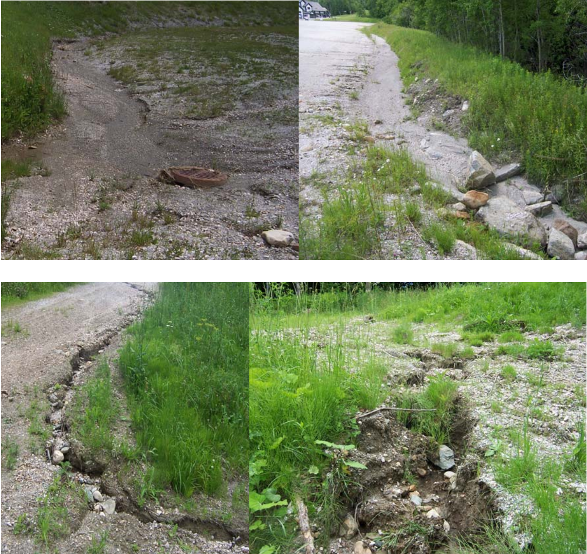
Photographs 36, 37, 38 and 39: These are several unstable and eroding swales overloading sediment to the Ram's Head stormwater basin from the Ram's Head parking lot (Photos 36 and 37) and basin access road (Photos 38 and 39).
