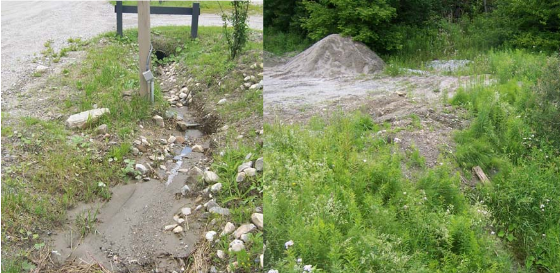
Photographs 40 and 41: Instable swale in the Mountain Green gravel parking lot and uncontained gravel/sand mound in north corner of parking lot – both conveying sediment to the Pinnacle Condo roadside swale (Photo 42).
