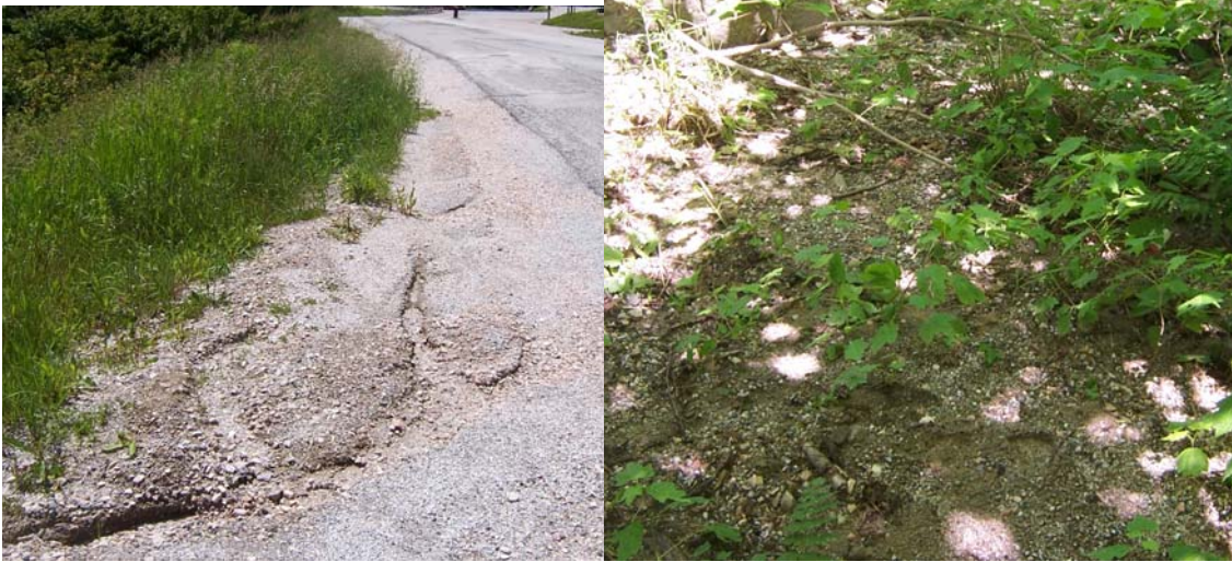
Photographs 25 and 26: There is eroding gravel off of the Gondola Road shoulder and into the riparian buffer of Roaring Brook.
