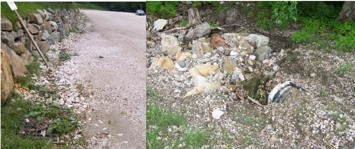
Photograph 45 and 46: The upper Whiffle Tree condo gravel parking lot (Photo 45) conveys sediment into a tributary of Roaring Brook via a storm drain. The outlet of the storm drain culvert is instable and eroding (Photo 46).
