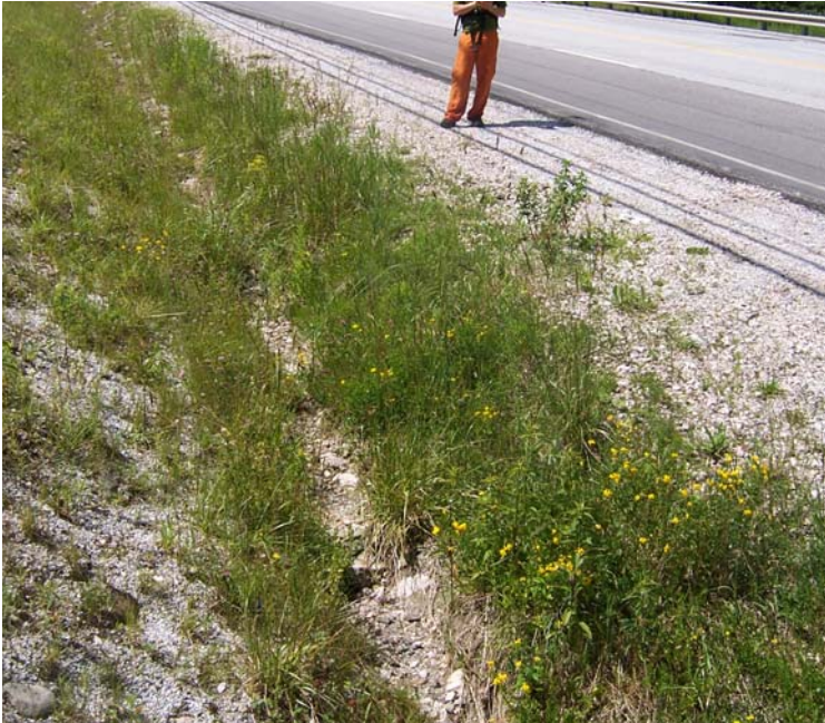
Photograph 18: A roadside swale along the east side of the access road is conveying fine sediment and gravel into a tributary of Roaring Brook.
