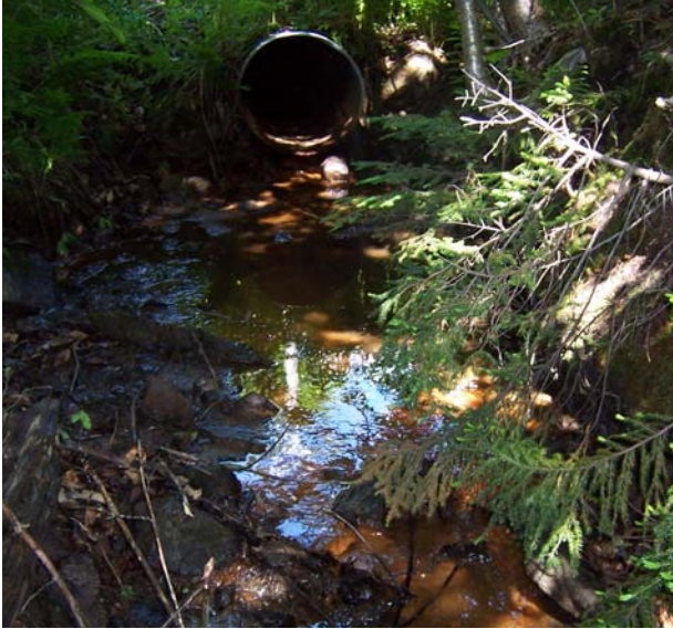
Photograph 13: The outlet from the sediment basin from the “E” and “F” parking lots has a rusted out culvert causing iron seepage and a sediment input into a small tributary of Roaring Brook.
