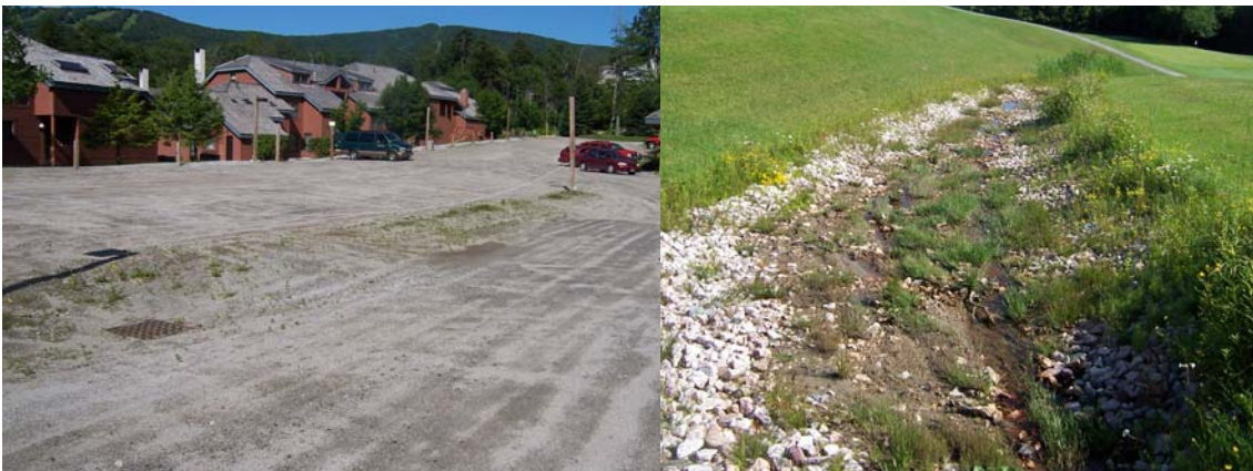
Photographs 3 and 4: Through a linked system of storm drains, culverts and swales, the unpaved parking lot at Trail Creek Condo Development is conveying sediment into a tributary of the East Branch of Roaring Brook.
