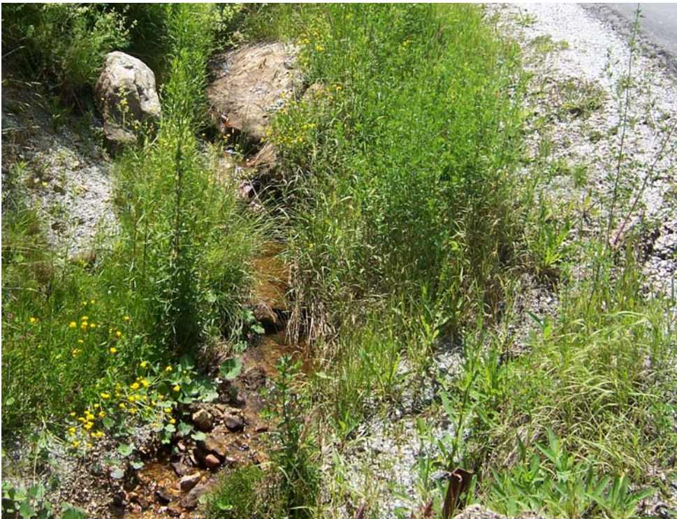
Photograph 33: Instable and eroding roadside swale US of culvert "C-40" on the east side of the Access Road.
