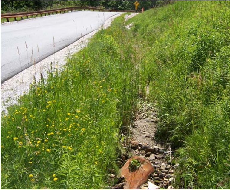
Photograph 28: Swale conveying sediment needs stone and check dams extended down to culvert “C-36”.
