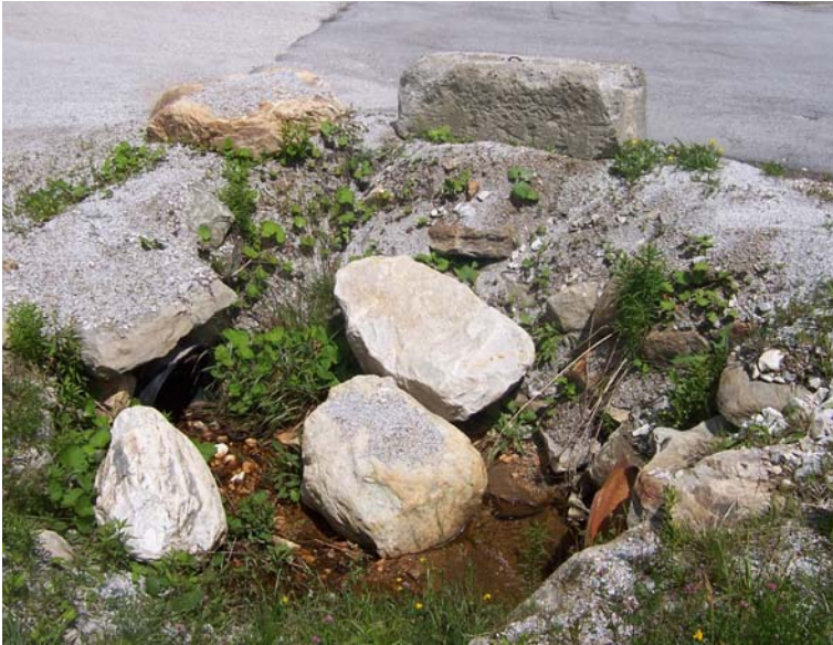
Photograph 34: Gravel is being washed into the day-lighted section of culvert "C-40".
