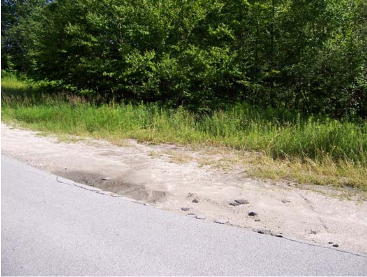
Photograph 5: Gravel run off from the edge of E. Mountain Road is contributing sediment to the East Branch of Roaring Brook around the outlet of culvert “C-77”.
