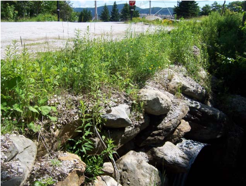
Photograph 12: Gravel from the parking lot above the culvert “C-22” inlet is conveying sediment into Roaring Brook over the boulder headwall.
