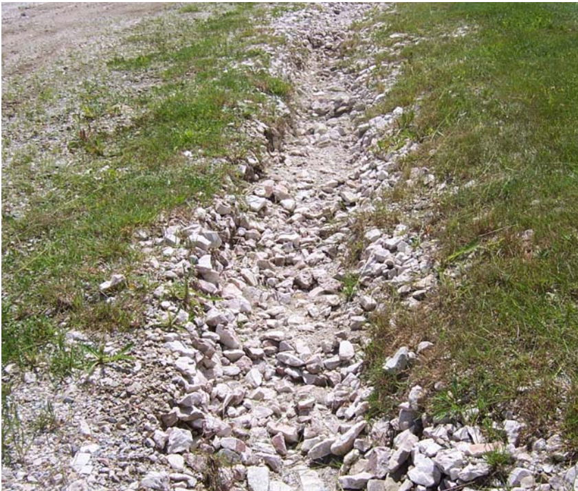
Photograph 27: There is an eroding swale located in the Gondola parking lot.
