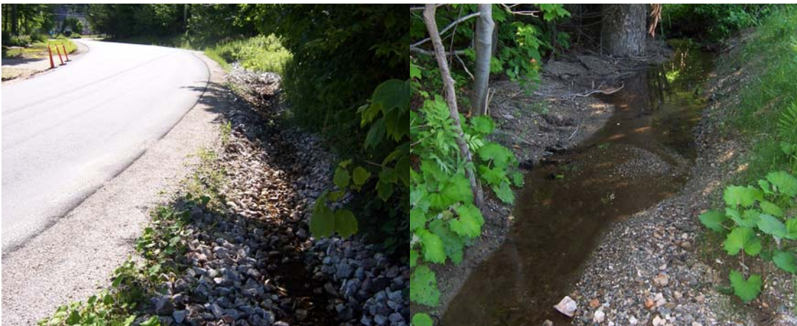
Photographs 6 and 7: Across the entrance of “Whiffle Tree” on the south side of E. Mountain Road, a roadside swale is conveying sediment into the East Branch of Roaring Brook.
