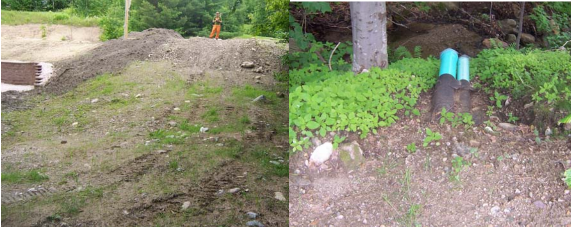
Photograph 47 and 48: The uncontained temporary soil disturbances in the lower Whiffle Tree Condo parking lot is conveying sediment to a tributary of Roaring Brook at the culvert outlet (Photograph 48).
