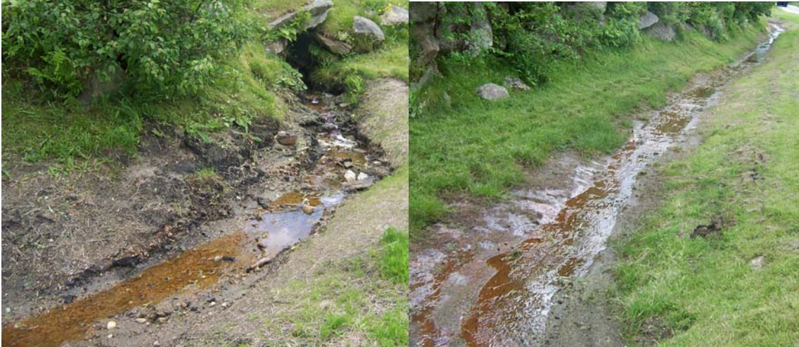
Photographs 43 and 44: The instable and eroding swale along Water Treatment dirt Access Road.
