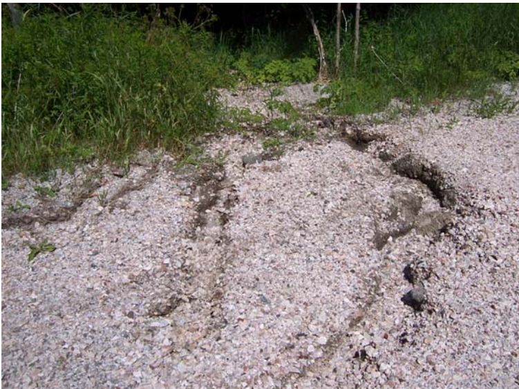
Photograph 17: Gravel is eroding off of a roadside bank down towards Roaring Brook on the west side of the access road.
