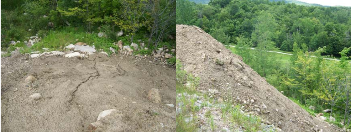
Photograph 1 and 2: Large pile (~40 ft high) of exposed and uncontained dirt in close proximity of a tributary of the East Branch of Roaring Brook. The pile of dirt is located at the northern end of the Lower Whiffle Tree lot and is actively eroding.
