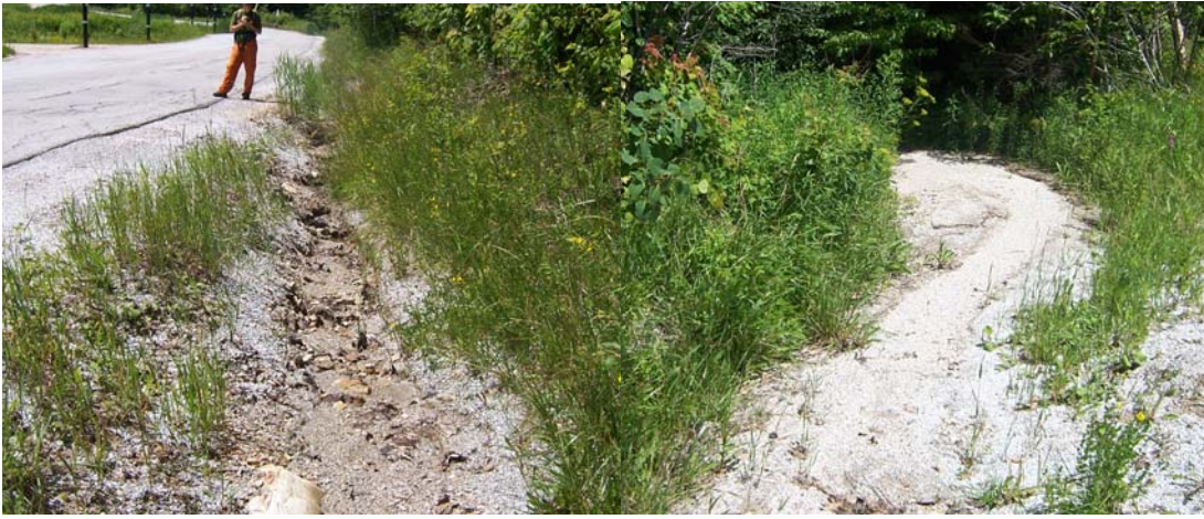
Photograph 31 and 32: Swale by "E" and "F" is instable and contributing gravel to the riparian buffer of Ram's Head Brook on river right.
