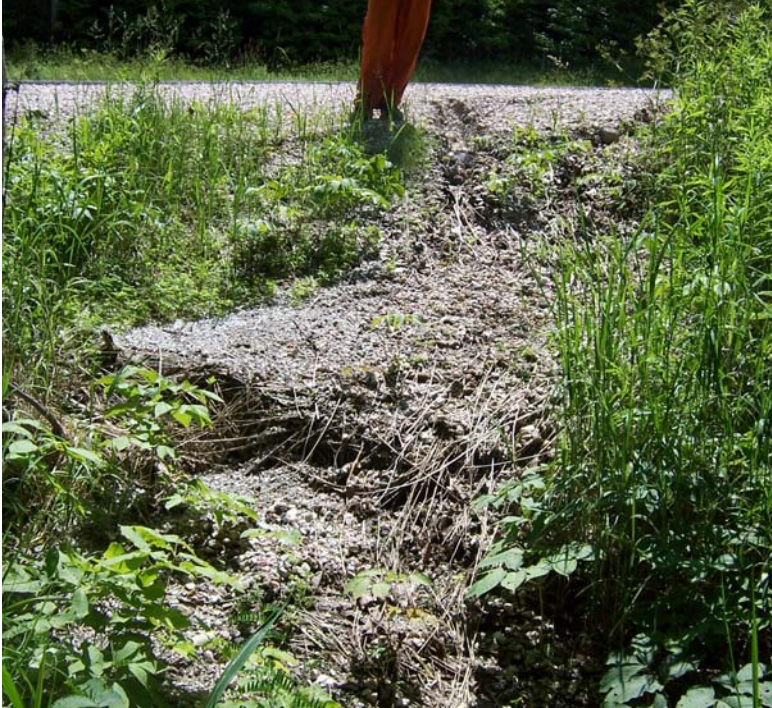
Photograph 16: Roadside gravel on the west side of the access road is washing down towards Roaring Brook.
