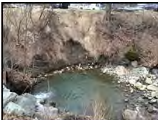
Trib. 3 slope failure at maintenance area (04/28/2014)
