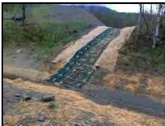
Gully repaired with RECP (05/22/2014)
