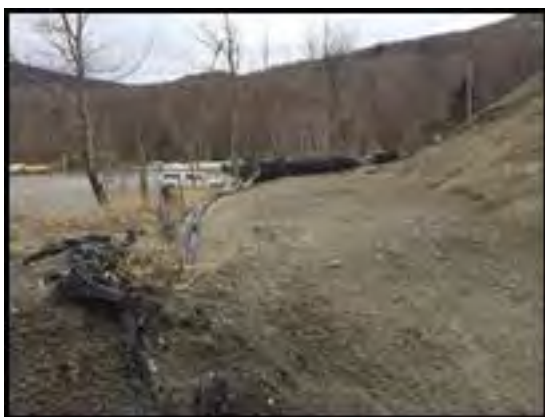
Overtopped silt fence at sand pile (04/28/2014)
