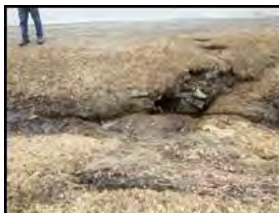
Slumped banks and clogged culvert inlet (04/28/2014)
