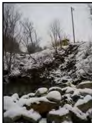
Trib. 3 slope failure at maintenance area (05/02/2012)
