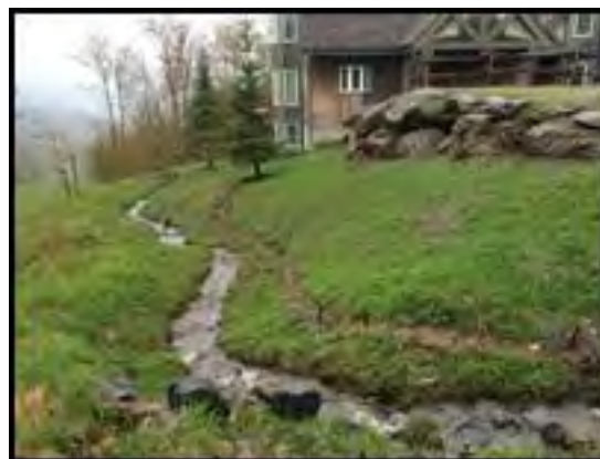
Straw wattle used to trap sediment (05/22/2014)
