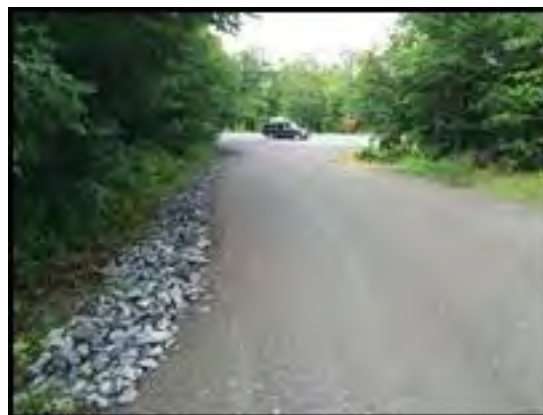
Regraded road with stone edging (08/07/2014)
