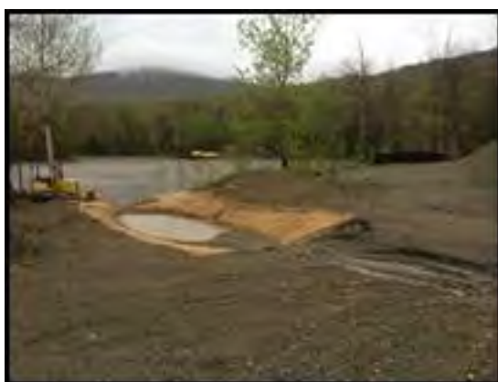
Temporary sedimentation basin at sand pile (05/22/2014)
