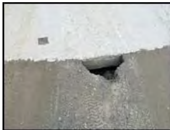
Eroded bridge approaches over Jay Branch (4/28/2014)
