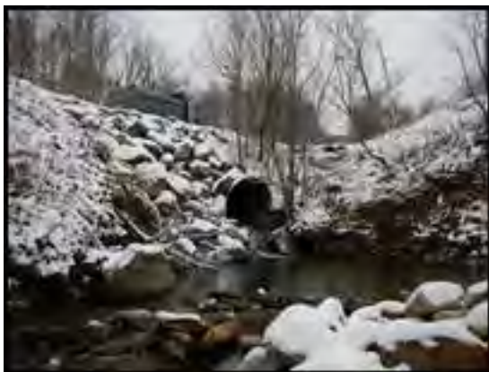
Undersized culvert at Stateside Road (11/08/2012)
