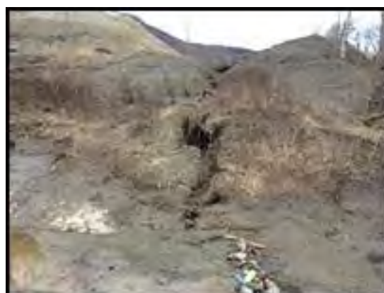
Slope erosion at Rt. 242 Parking Lot (04/28/2014)
