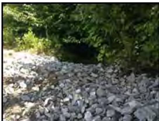
Channel regraded and transition stabilized (07/17/2014)
