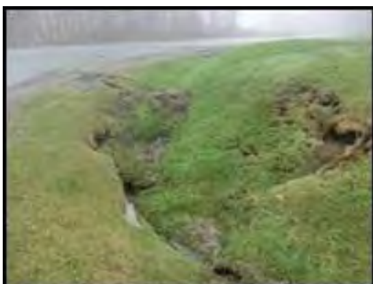
Slumped banks and clogged culvert inlet (05/02/2012)
