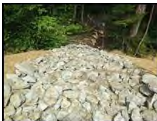
Rip rap outlet spillway (08/20/2014)
