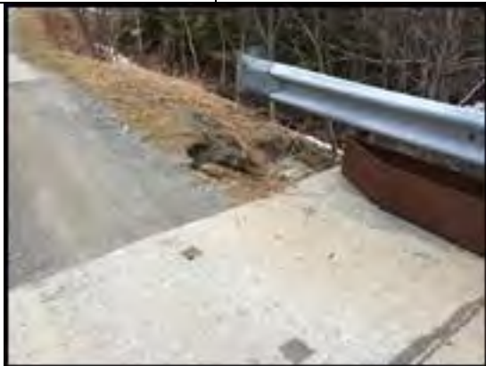
Eroded bridge approaches over Jay Branch (04/28/2014)
