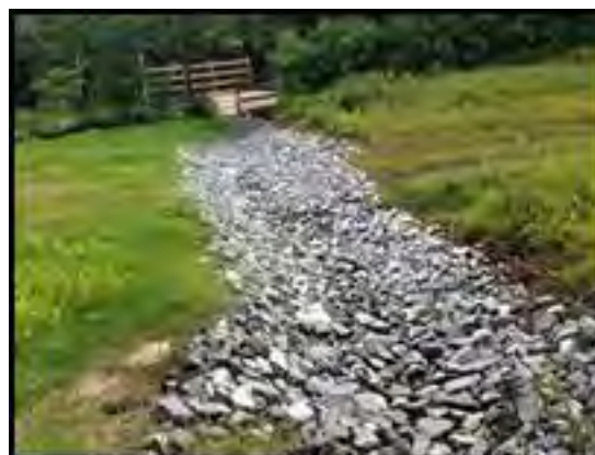
Stabilized waterbar looking downhill (08/19/2014)
