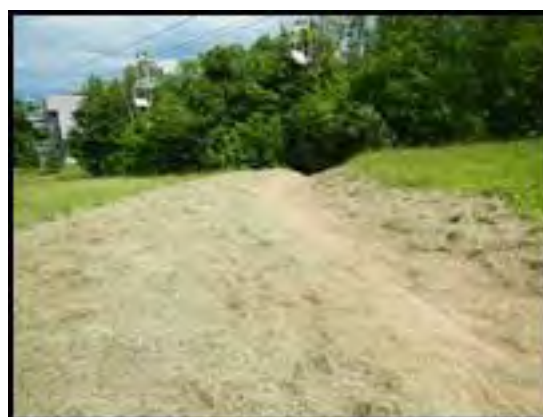
Regraded and stabilized water bar crossing (07/09/2014)
