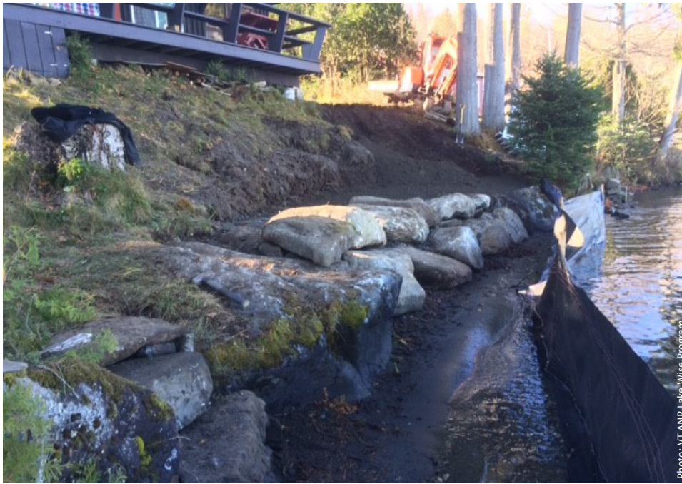
Before (left) and after (right) regrading and installation of a stone toe to protect this bank.
