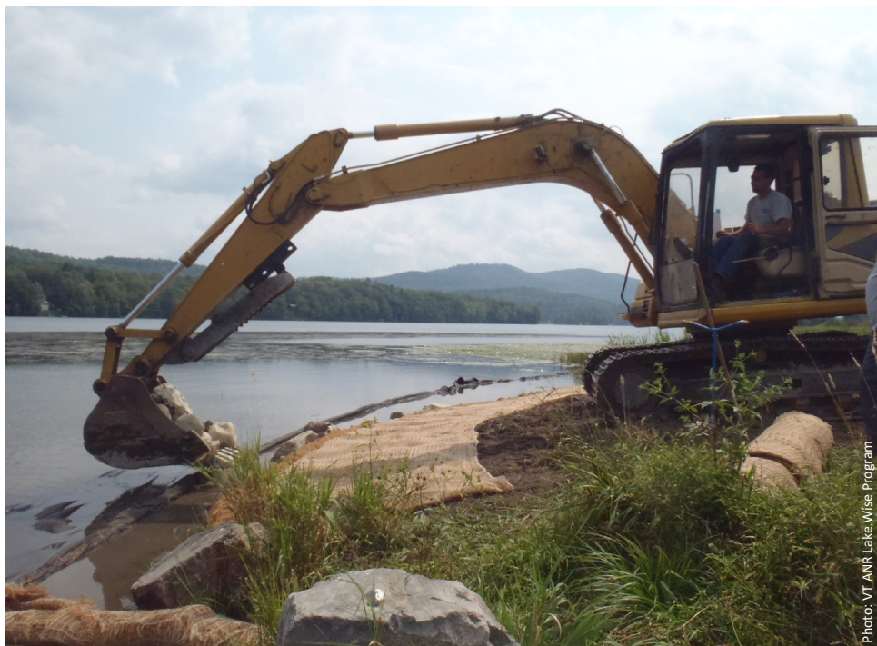
A stone toe is installed along the Lake Iroquois shoreline in Williston, VT to stabilize the banks. Erosion control blankets were installed after the slope was regraded and native vegetation will be installed.
