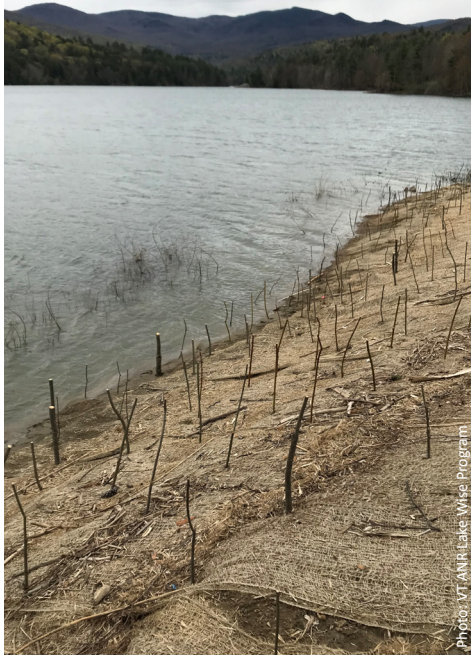
Live stakes (left) and live fascines (right) can be used to stabilize slopes. Note that the live fascine photo was taken directly after installation and additional soil stabilization was also completed.
