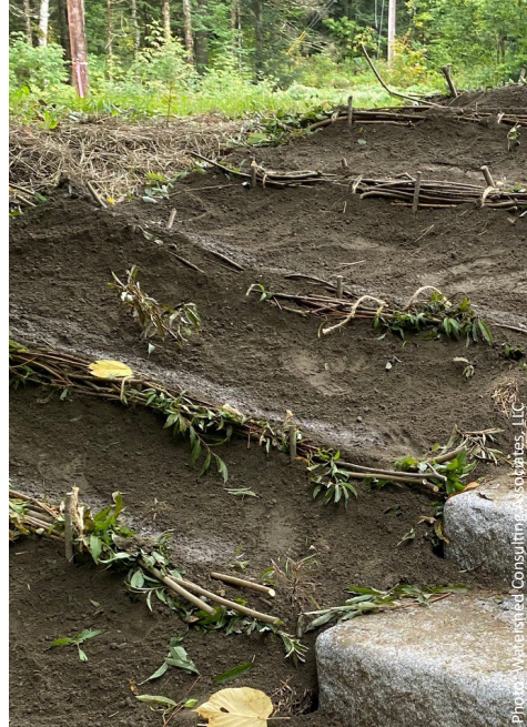
Live stakes (left) and live fascines (right) can be used to stabilize slopes. Note that the live fascine photo was taken directly after installation and additional soil stabilization was also completed.
