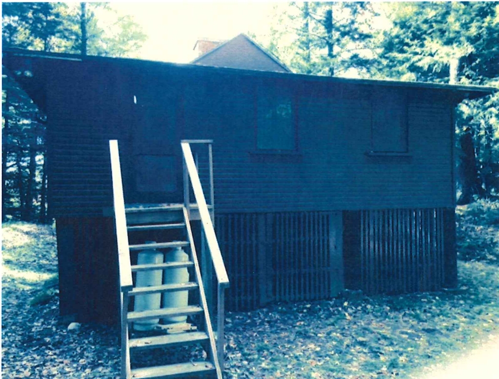
Perspective 2: View of camp from driveway (facing West)
