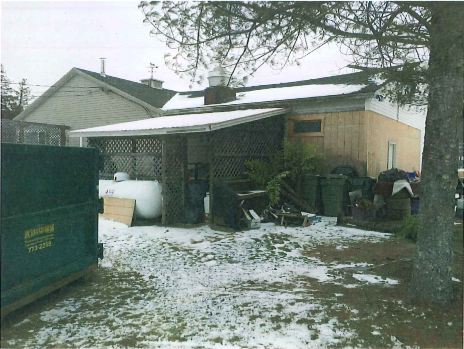
View northeast of restaurant building's side and shed. This is the location of the kitchen addition.
