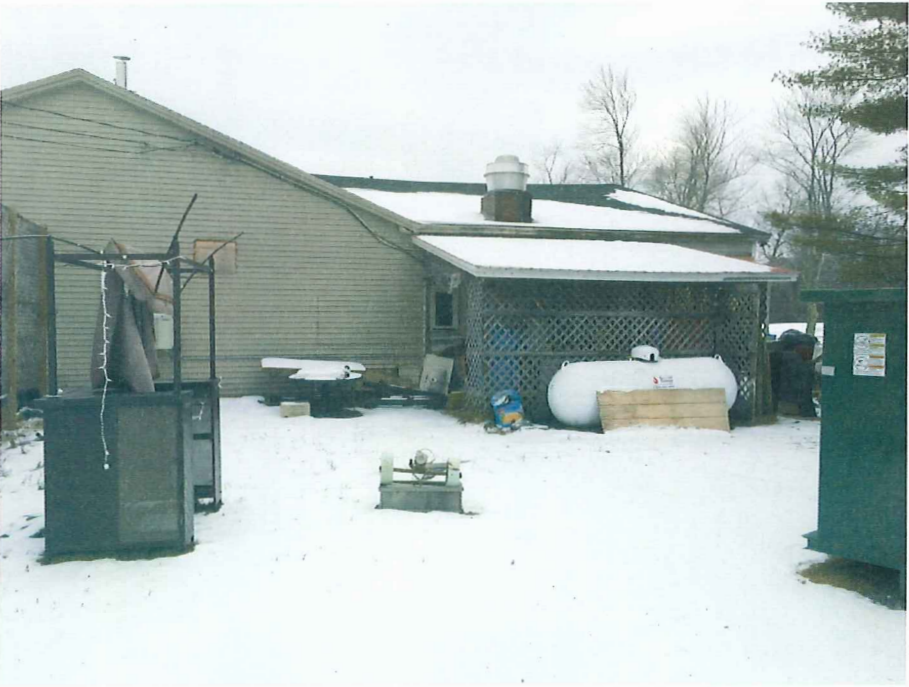
View east of restaurant building's side and shed. This is the location of the kitchen addition.
