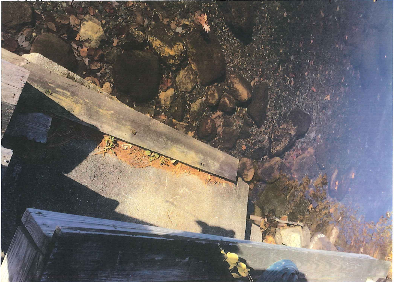
McNARYWAY ↓ CONCRETE FOOTER, IN LAKE, EXISTING, TO BE REMOVED.
