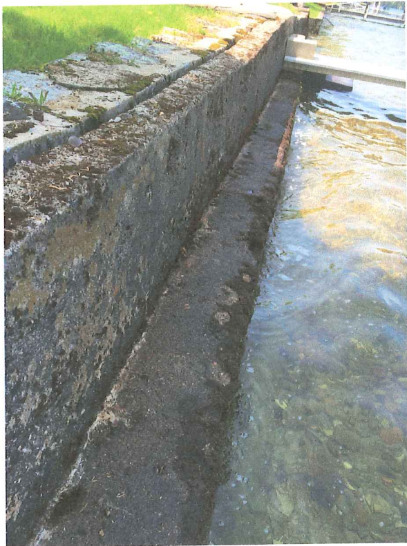
Picture showing overall condition of wall
