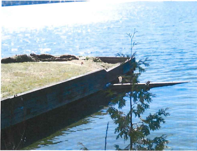
North side of dock
