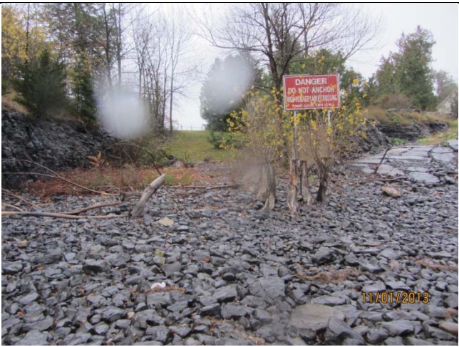
Photograph 4. From Lake Champlain shoreline, looking east. Existing submarine cables are buried from sign to Terminal Station.
