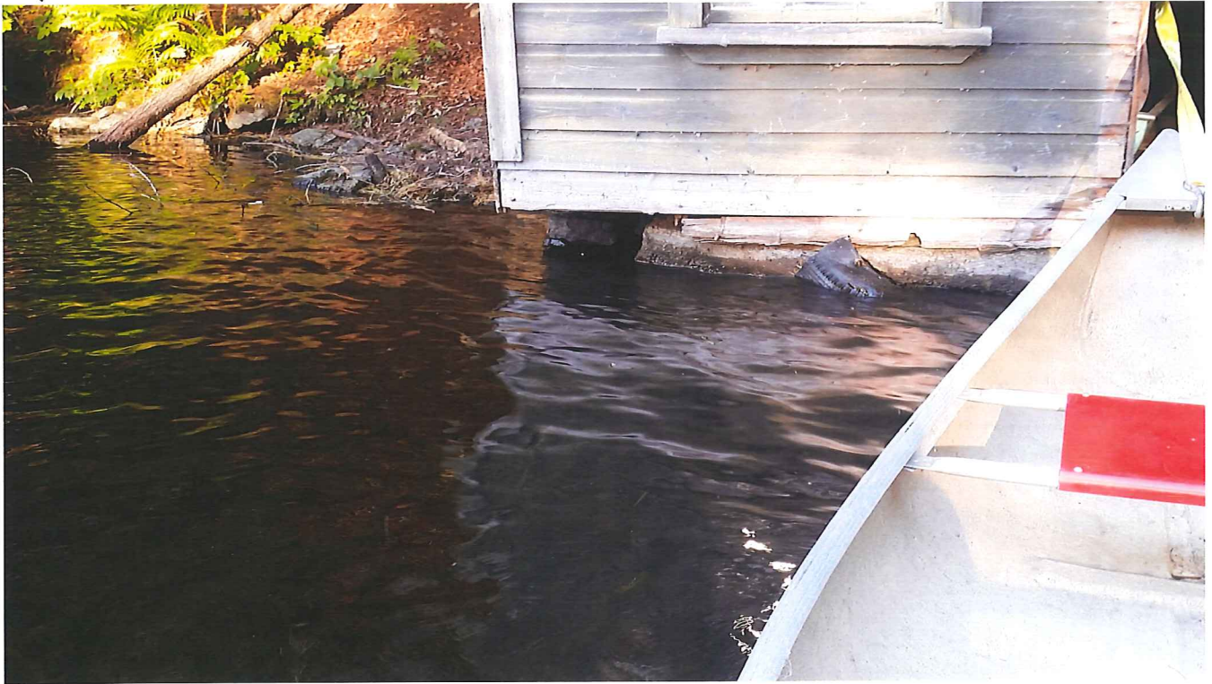
FRONT BOATHOUSE - FOUNDATION
