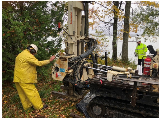
Figure 1. Installing a monitoring well to collect groundwater samples.
