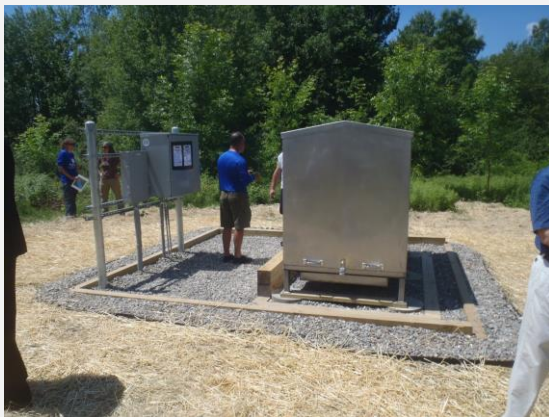
Figure 5. Lake Carmi aeration system compressor cabinet at Lake Carmi State Park (left) and bubbles produced in the lake by the aeration system during operation (right).
