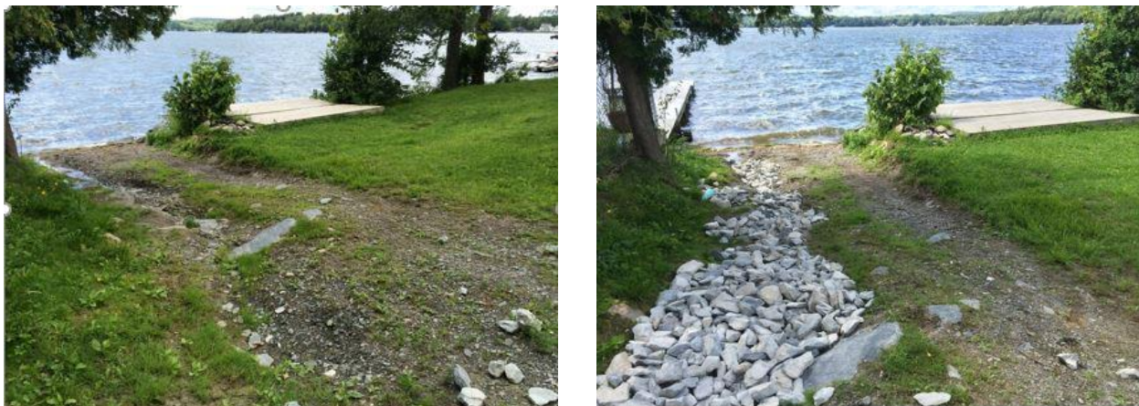
Figure 7. Before (left) and after (right) stabilization of an eroding lakeshore access path to Lake Carmi, completed by the Franklin Watershed Committee as part of the Lake Wise Program with funding from DEC’s Clean Water Initiative Program.
