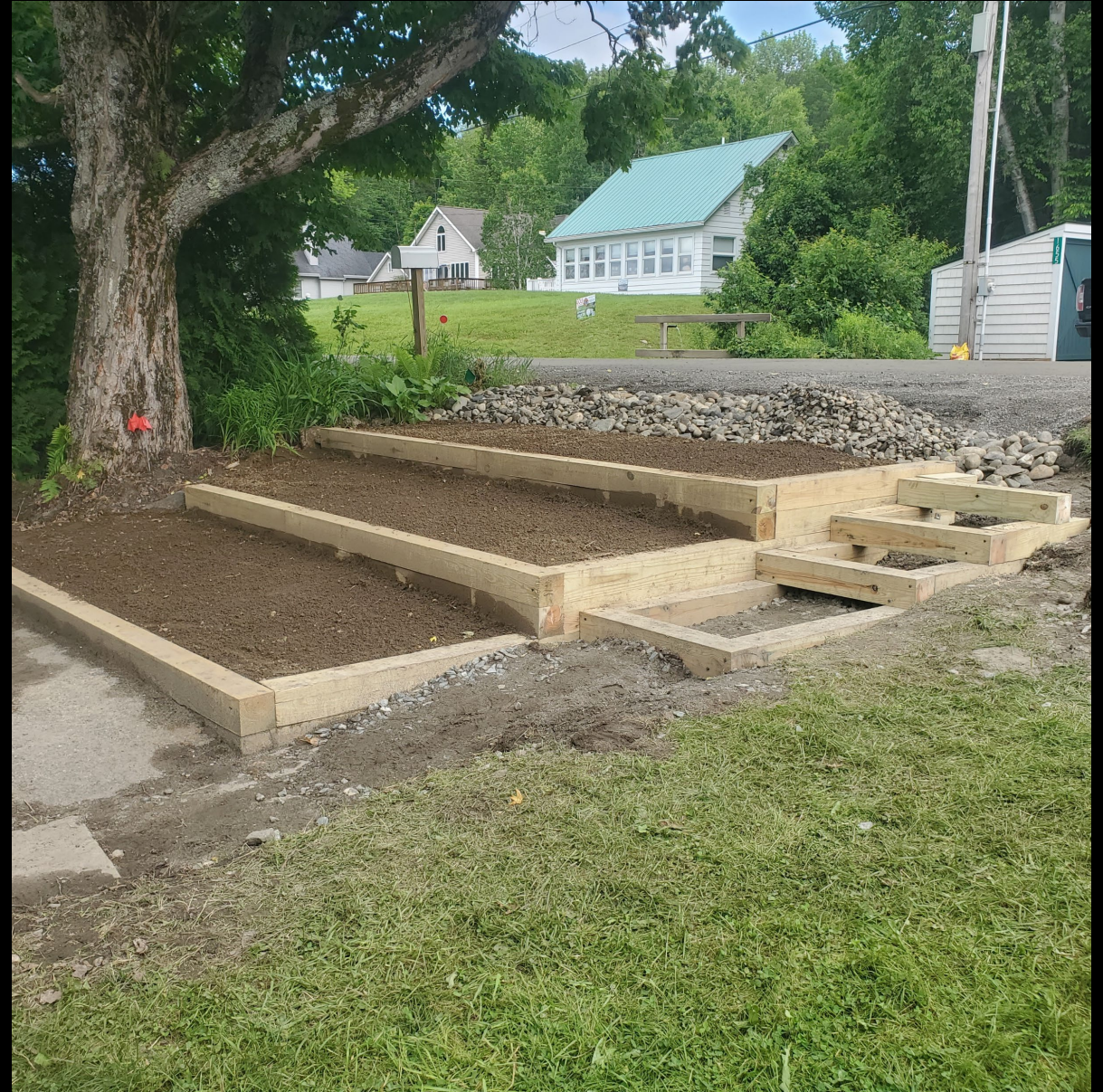
...and another 6" of topsoil was placed for planting media.
