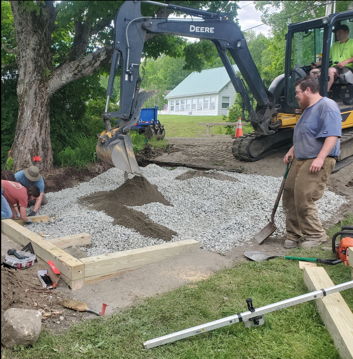
...then backfilled with 24" drainage stone & 6" septic sand.
