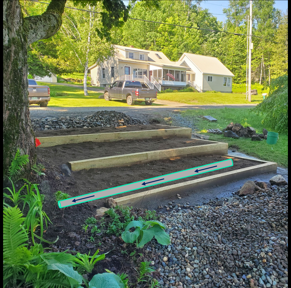
...and an underdrain lies beneath the infiltration bed.
