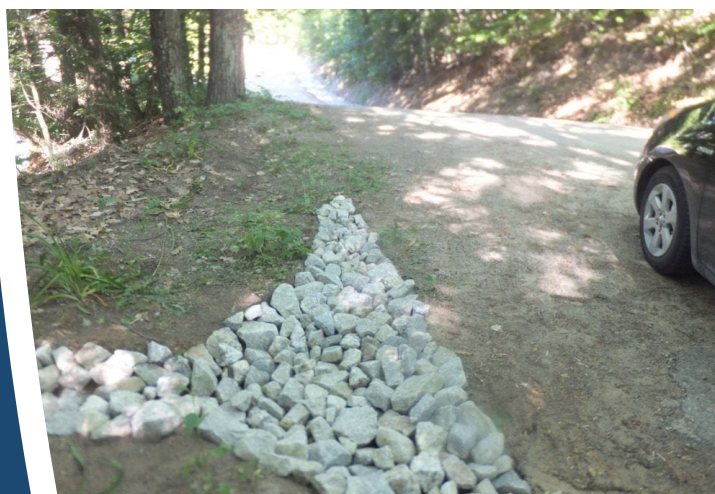
Turnout stabilized with angular rock .
