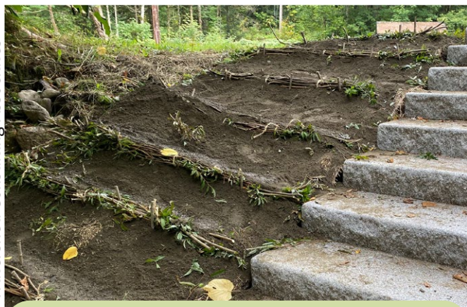
Section of a fascine > staked into a steep bank. Vermont Bioengineering Manual
