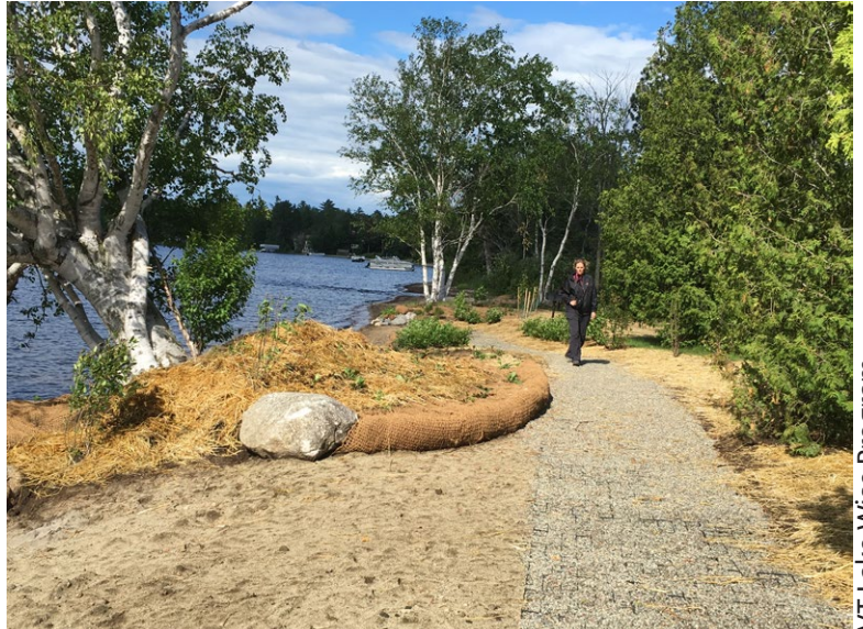
ADA compliant permeable geogrid and peastone pathway.
