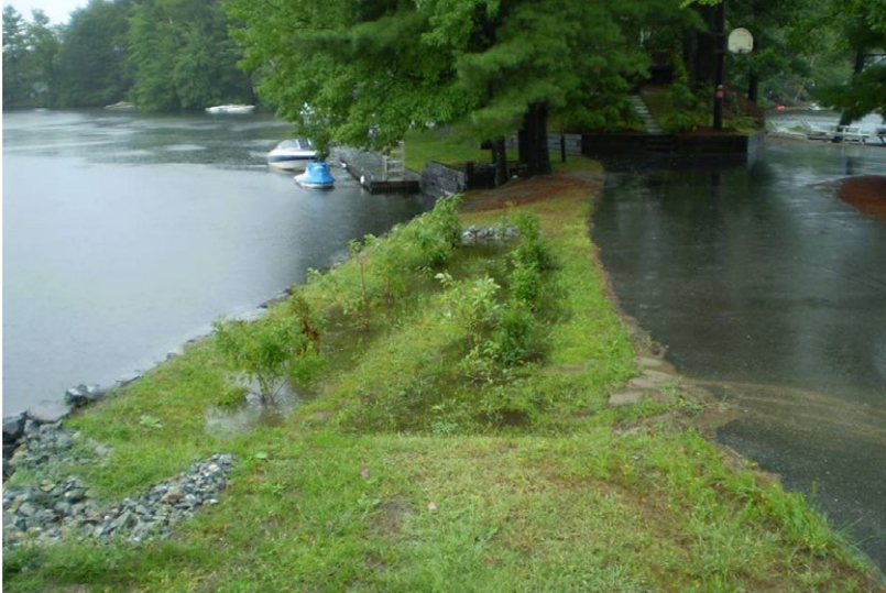
A vegetated swale at Lake Shirley, MA and open-top culverts at Lake Eden F&W Access intercept road runoff.
