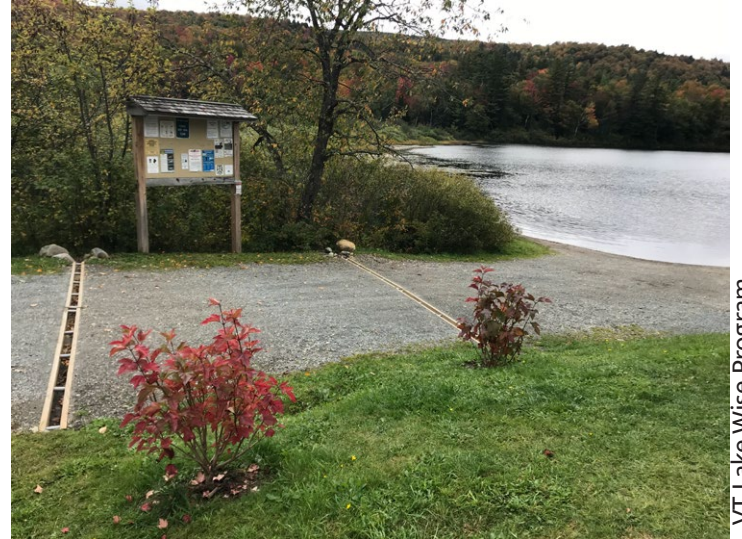
A vegetated swale at Lake Shirley, MA and open-top culverts at Lake Eden F&W Access intercept road runoff.
