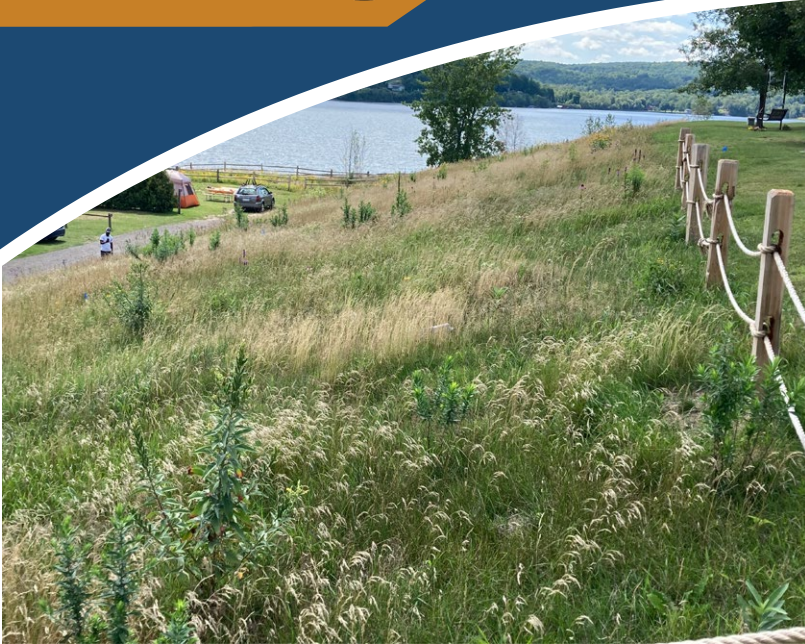
An upland meadow and rain garden slow down and soak up stormwater at steeply sloped Prouty Beach in Newport.
