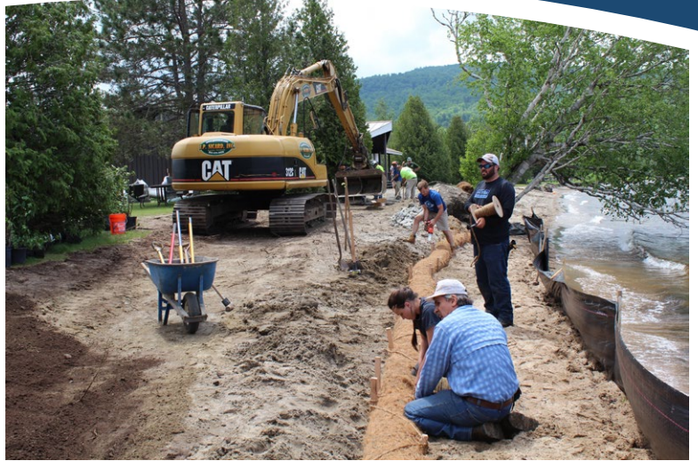
INSTALLATION. Erosion control with fiber coir rolls.
