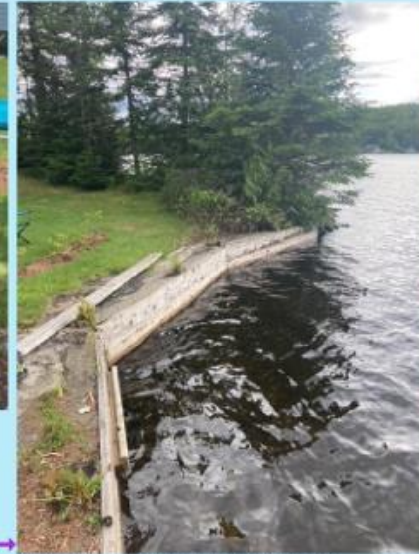
View of retaining wall from north side
