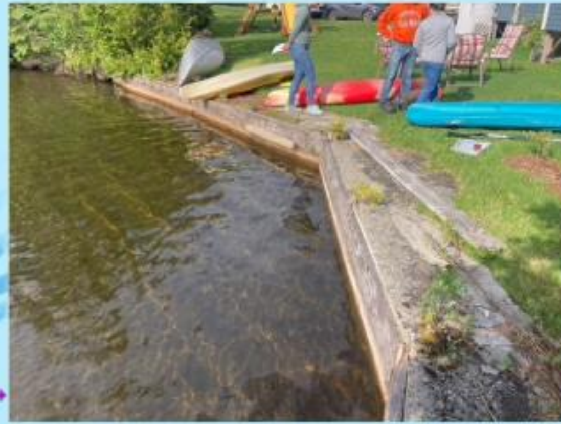
View of retaining wall from south side
