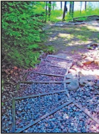
**Note:** Infiltration steps may not require side timbers, especially if the steps are in an eroded pathway where the surrounding land is higher. In this case, extend the timbers into the adjacent banks so water will not go around the steps.
