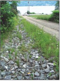
steep road that serves several camps with a rock lining installed to prevent the previous on-going erosion of the ditch.
