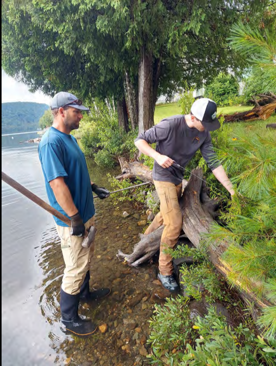
Driving duckbill anchors & cabling the rootwads & logs
