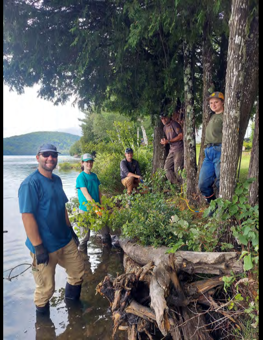
Logs are also interlocked between rootwads & existing cedars
