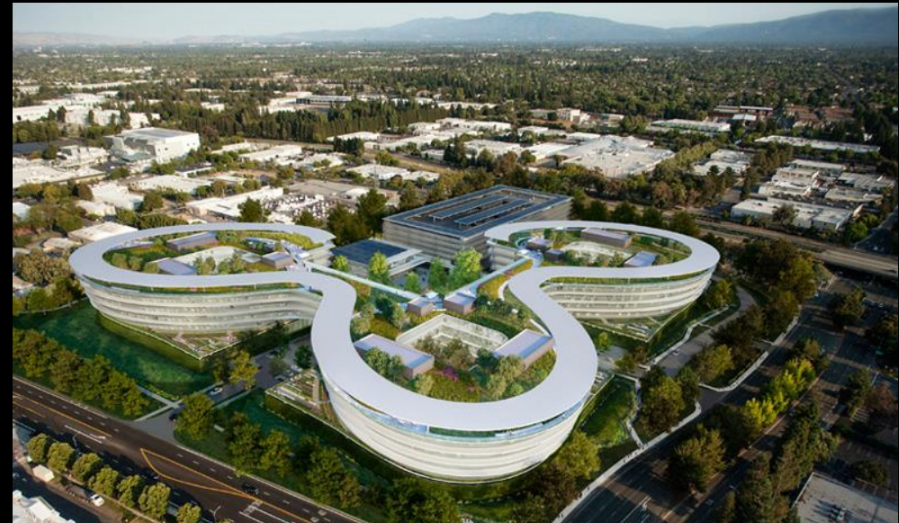
Apple 3 LEED-Platinum office in Santa Clara, CA
